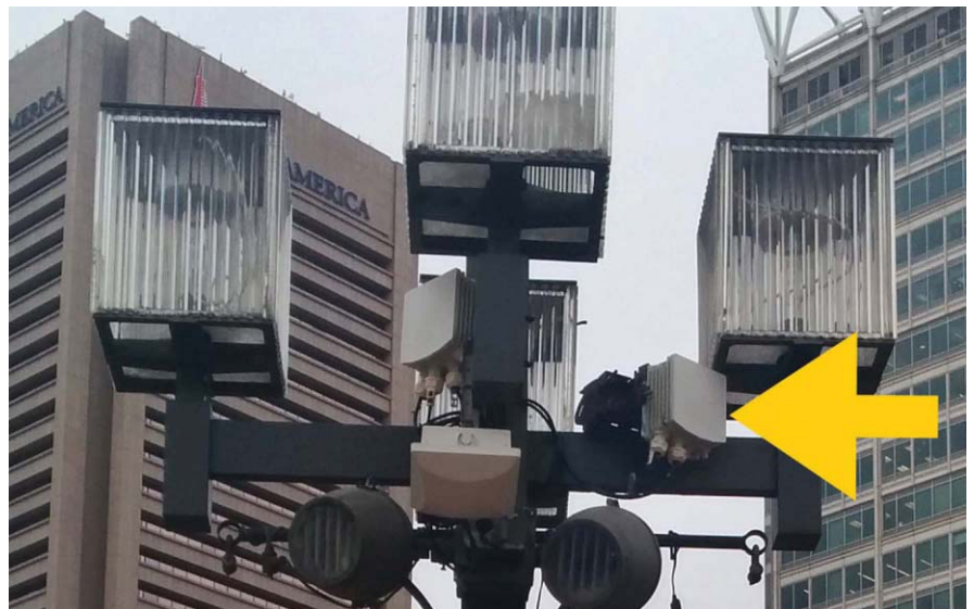
A lamppost in Baltimore that supports an access point for the city's free Wi-Fi at the historic Inner Harbor. Above: A 60-GHz EtherHaul-600T backhaul radio made by Siklu is small enough to be hardly noticeable. Millimeter-wave technology combines high throughput and low interference for a high level of network capacity.
