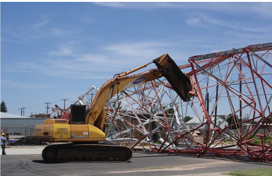
On June 26, 2007, a high wind felled a 300-foot tower in Seminole, Texas. It damaged the roof of the Agape Church and crushed the church's bus. Photos by Ron Robinson
