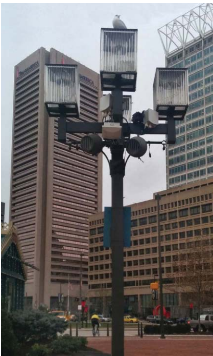
A lamppost in Baltimore that supports an access point for the city's free Wi-Fi at the historic Inner Harbor. Above: A 60-GHz EtherHaul-600T backhaul radio made by Siklu is small enough to be hardly noticeable. Millimeter-wave technology combines high throughput and low interference for a high level of network capacity.
