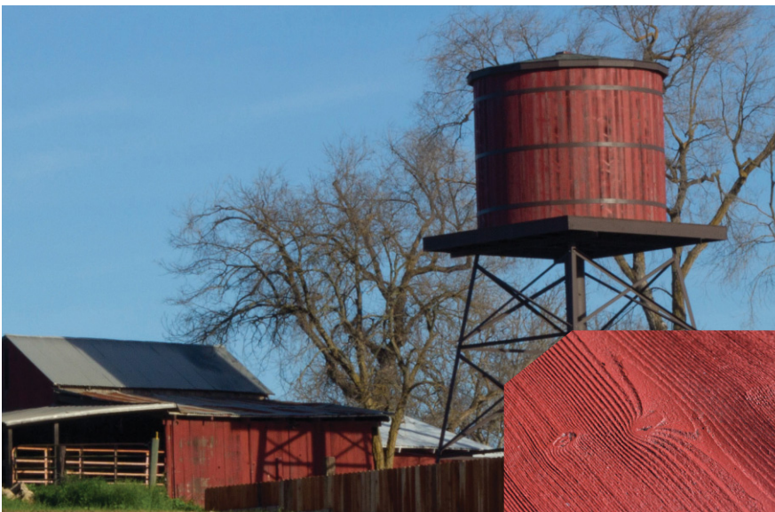
A rustic western water tank has aerospace-grade panels, custom-formed to duplicate weathered wood and to match an old barn. Inset: A close-up of the grain detail in the fiberglass-reinforced panel.
