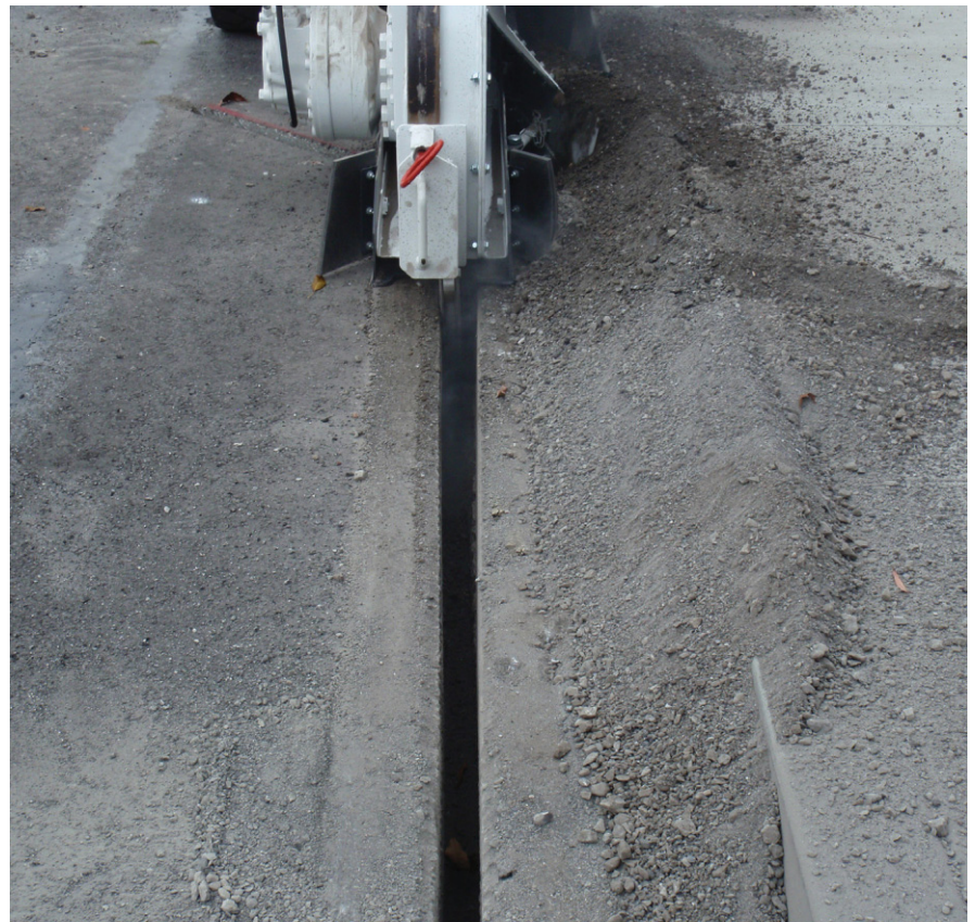
Instead of the 1-foot-wide to 2-foot-wide trench needed for a traditional inner duct, a microduct uses a microtrench an inch or two wide. The manhole need not be excavated for access, and no plating is needed for vehicular crossing.
