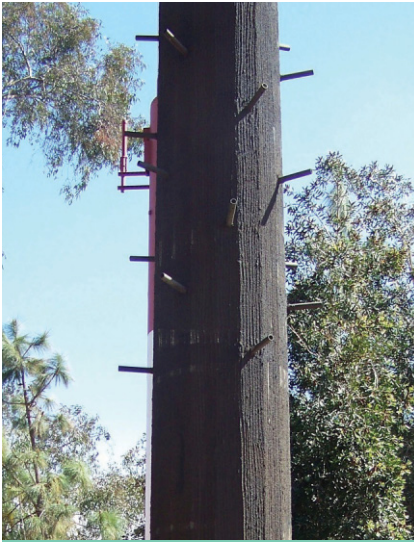
This is about as cheap as bark can get – use a tile trowel to spread stucco on a pole.
