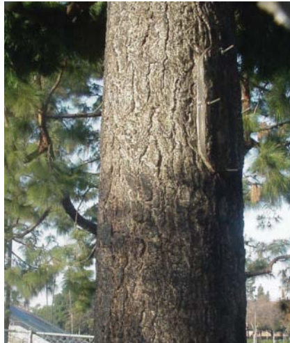
When realism is important, this is the best bark available. It is molded from real trees and then applied to the tower (and with newer processes, it holds up as well as any other bark).
