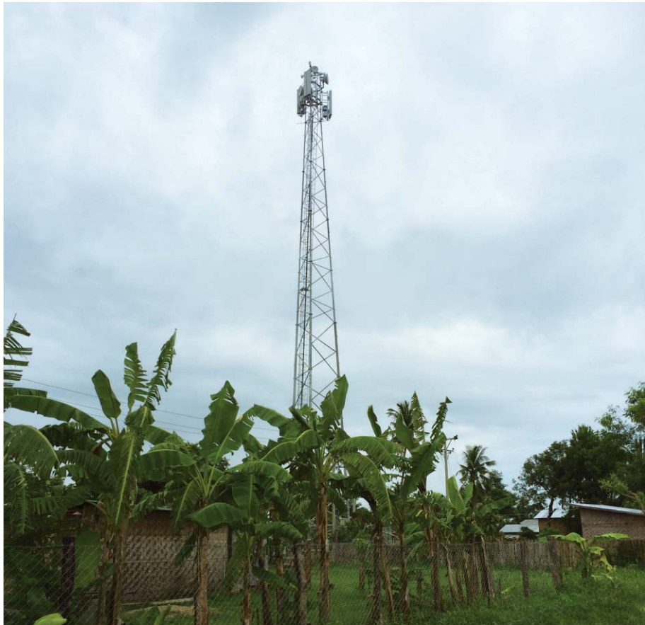
A rural site in Myanmar powered by Cummins generator sets.
