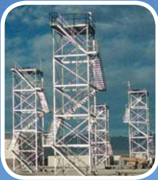
Creech Specialty Structure
