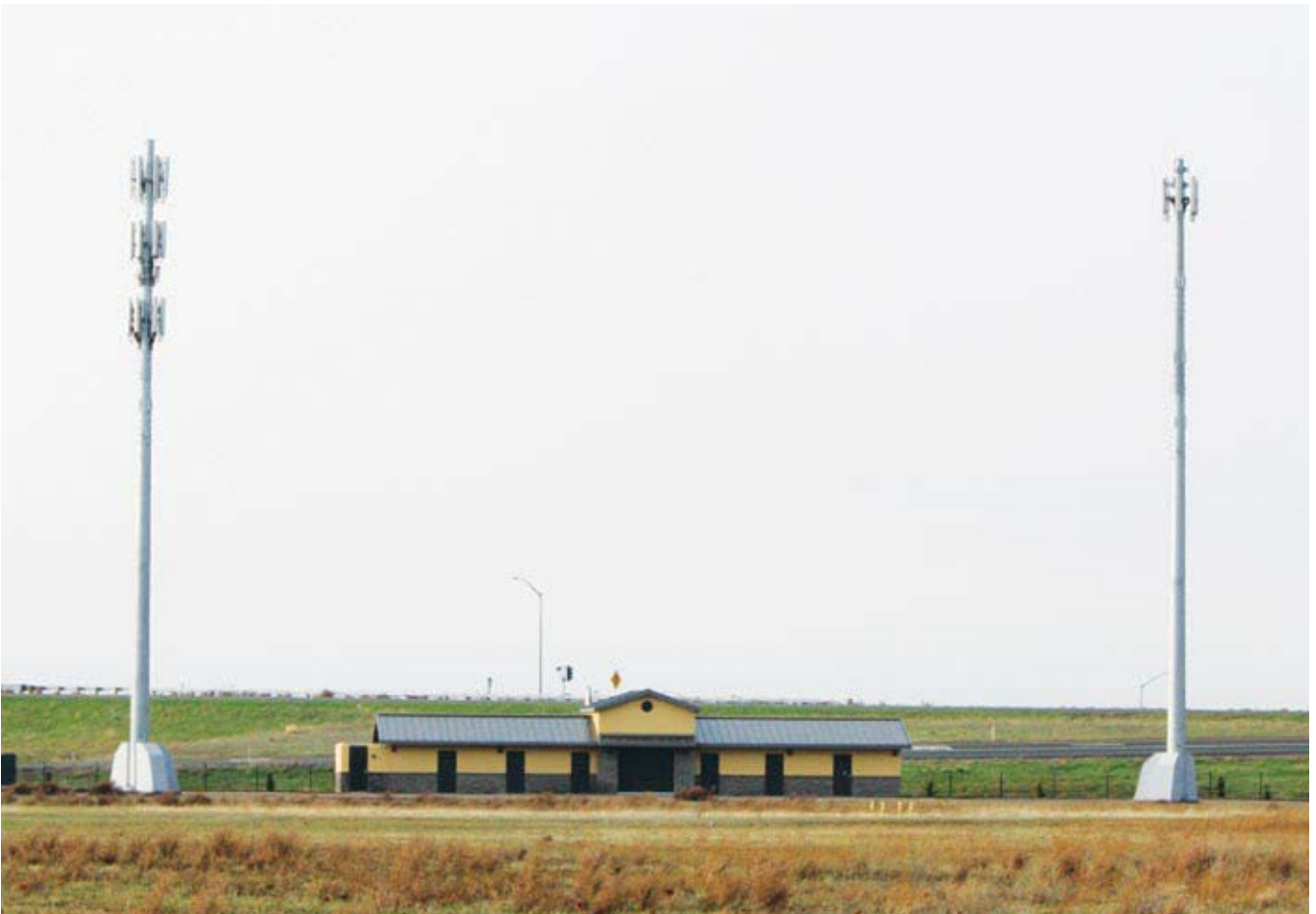
At the completed facility, the center room provides storage for the city's park maintenance equipment and public safety radio equipment. Three room spaces to each side of the center room are reserved for the carriers' radio equipment. On the tower to the left, MetroPCS occupies the uppermost rad center and AT&T Mobility occupies two rad centers directly beneath. On the tower to the right, Verizon Wireless occupies the uppermost rad center.
