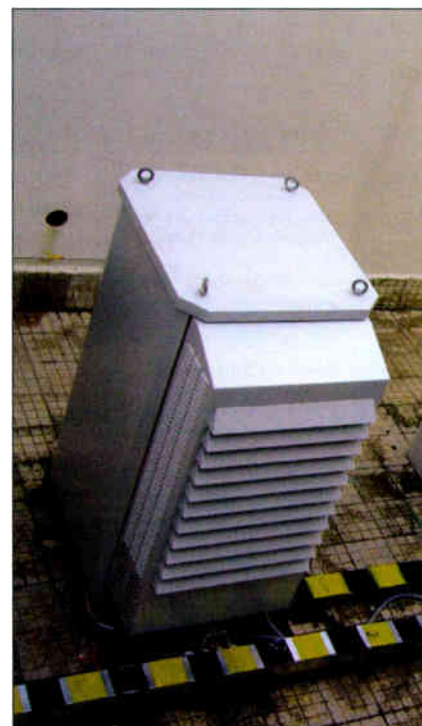
Dual integrated fuel cell systems provide extended-run backup power.
