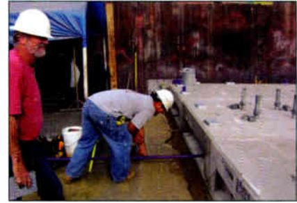
Workers install post-tensioning hardware and adjust the post tensioning to 50 percent.
