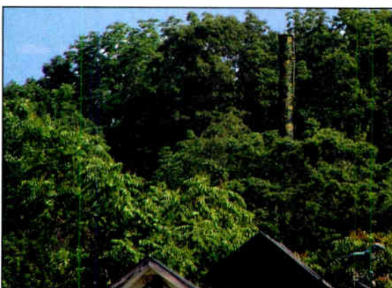
Invisible Towers' projects employ a number of camouflage solutions designed to engage community support for antenna sites.
