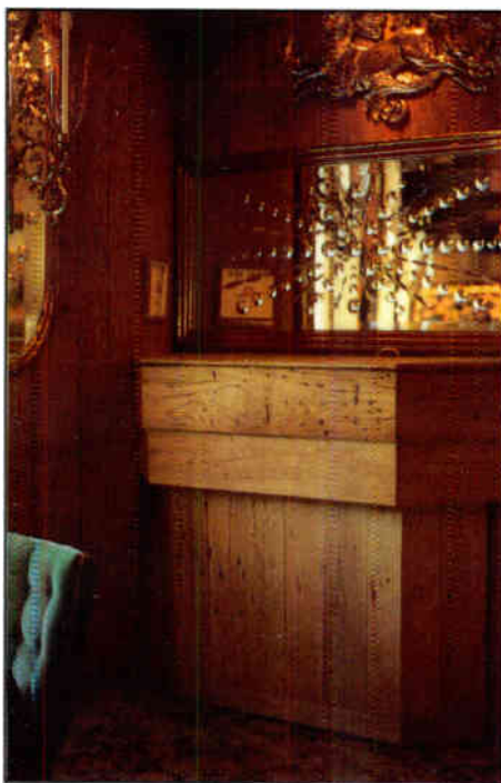
With the electronics racks' locking top in place, its chestnut exterior blends into the Chestnut Room's decor.
