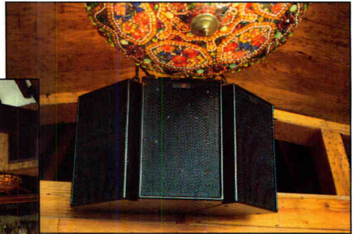
The Chestnut Room's main cluster of three EAW JF200i's just fit the space left by moving a large Tiffany chandelier.
