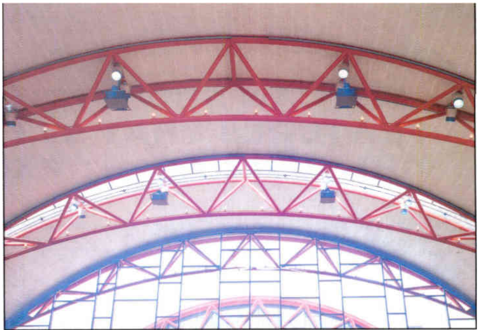
Eighteen cluster span these arches featuring Electro-Voice components.
