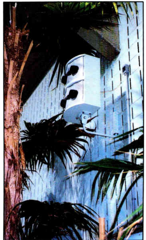
Three pairs of stacked Bose 802s were painted off site to match the back wall.
