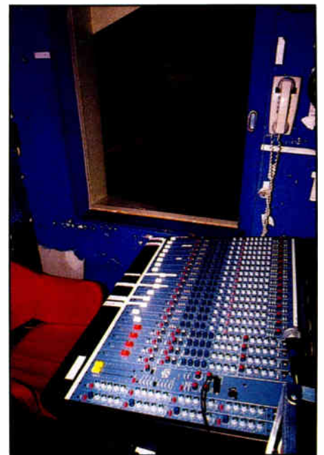
View of booth, mix positions.
