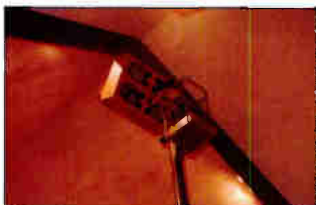
A special "Genie" lift was used to bring the cluster into position.
