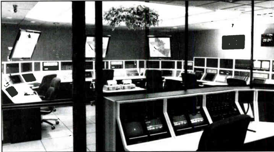
The command center underneath the headquarters building. This is where all police communications are routed and all emergency activities are coordinated.
