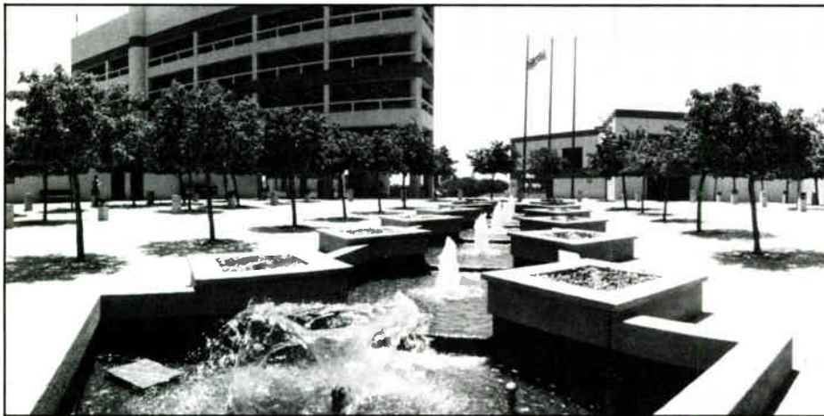
Police Department Headquarters, Huntington Beach, CA.
