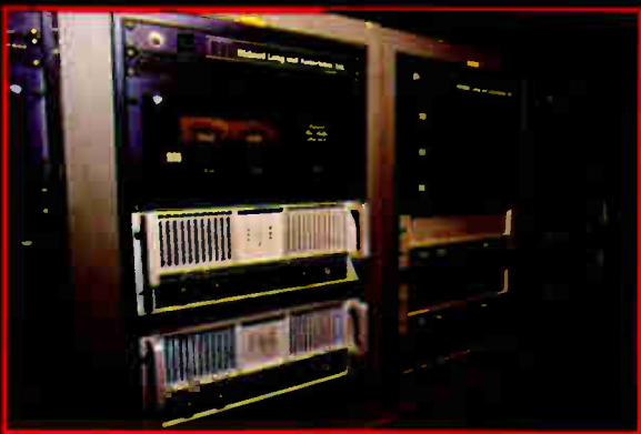
Maurice Brahm is the Underground's general manager. The club's six rack, 18 amp system, consists of seven BGW 750 Amps, four Crown D150 Amps, two Crown PS A-2 Amps, an RG Dynamics Expander, and two White 1/3 Octave Equalizers.
