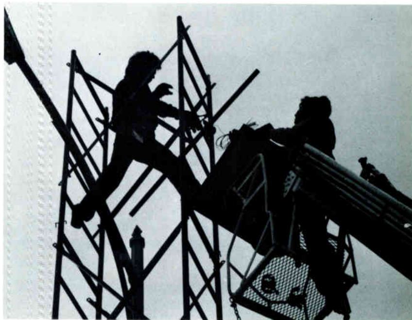
Installing the M4 loudspeakers.
