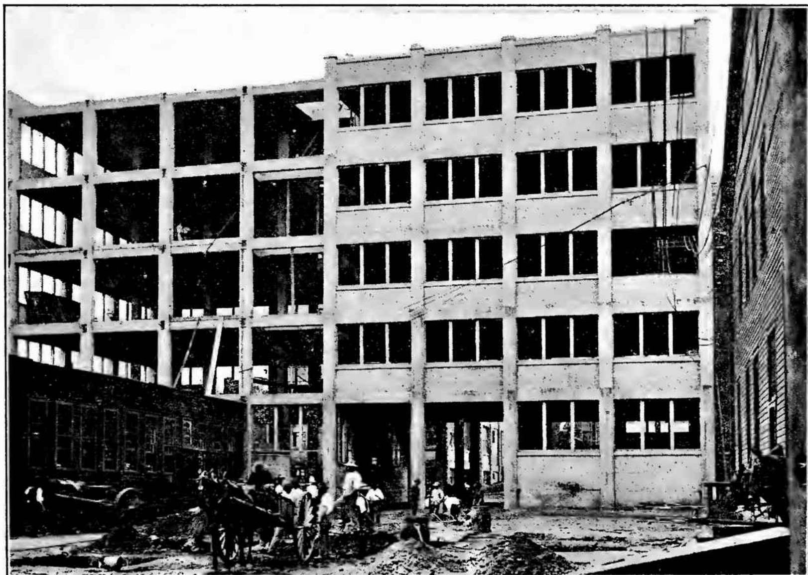
No. 2. NEW ADDITION TO No. 18, WOODWORKING AND CABINET BUILDING.
