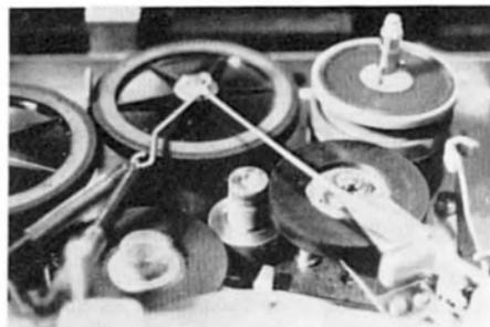
**Upper right:** Sony again but this time the machine is intended for horizontal or vertical operation. Take-up torque is necessarily stronger and setting can be difficult. The pulley rides up its spindle for fast-forward drive and the pulley angle is important.
