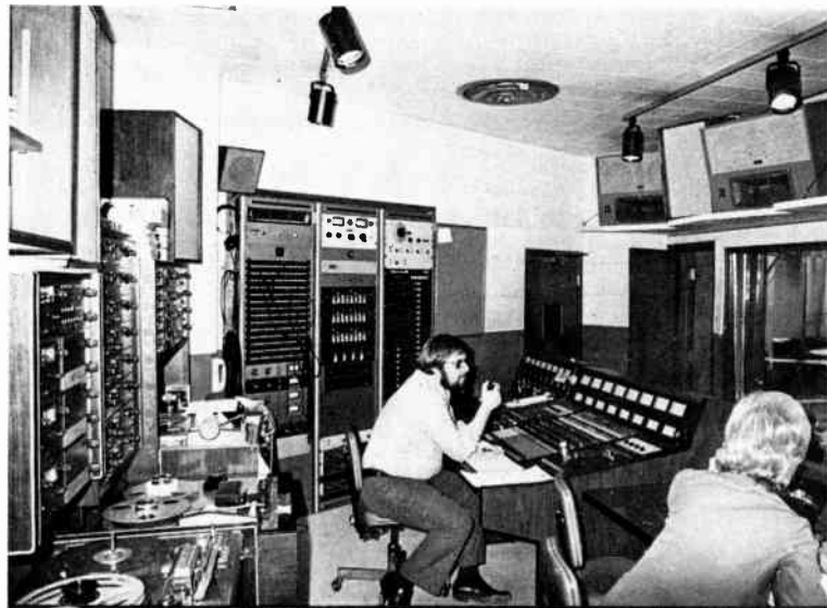
Overall view of the control room showing the location of monitor speakers and the elaborate mixing console.
