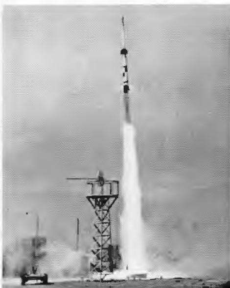
The first Ballistic Research Laboratories rocket firing to be a preliminary to IGY. This is a Nike-Cajun (the Nike as the booster and the Cajun for the second stage) launched at White Sands Proving Ground, N. M., on August 9, 1956. The Nike-Cajun is one of two types of rockets to be fired during IGY.
