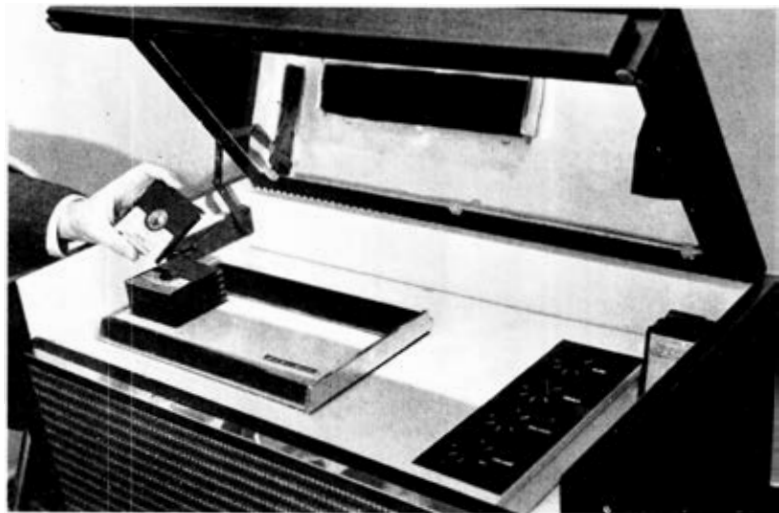
Above: Stereo tape carriage system developed in the CBS Laboratories in America—a strong candidate as the standard music reproduction system of the future. Below: The contemporary line—provision for disc, tape and radio is made in this long, low modern cabinet ( E. Gomme Ltd. ).
