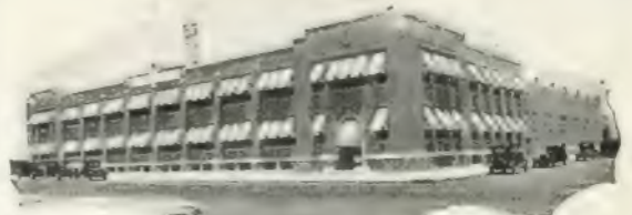
Philadelphia Plant of U. P. C. N. W. Cor. Chestnut and 56th Sts. Headquarters Chilton Class Journal Co.
