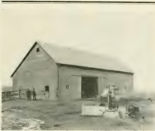
T HE Maurer barn was built in 1912. On the ground floor are stalls for fifteen cows and six horses. The "loft" above is filled with "roughage" and hay. In the foreground is the water-trough, into which a gasoline engine pumps water from one of two wells on the farm
