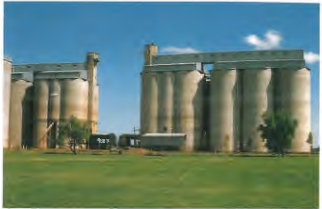
Silos for storing barley. Each silo is 40m high and holds 2500 tonnes of grain.
