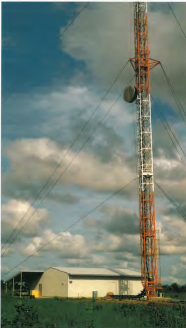
Mast torsional stabiliser at 45 m level.
