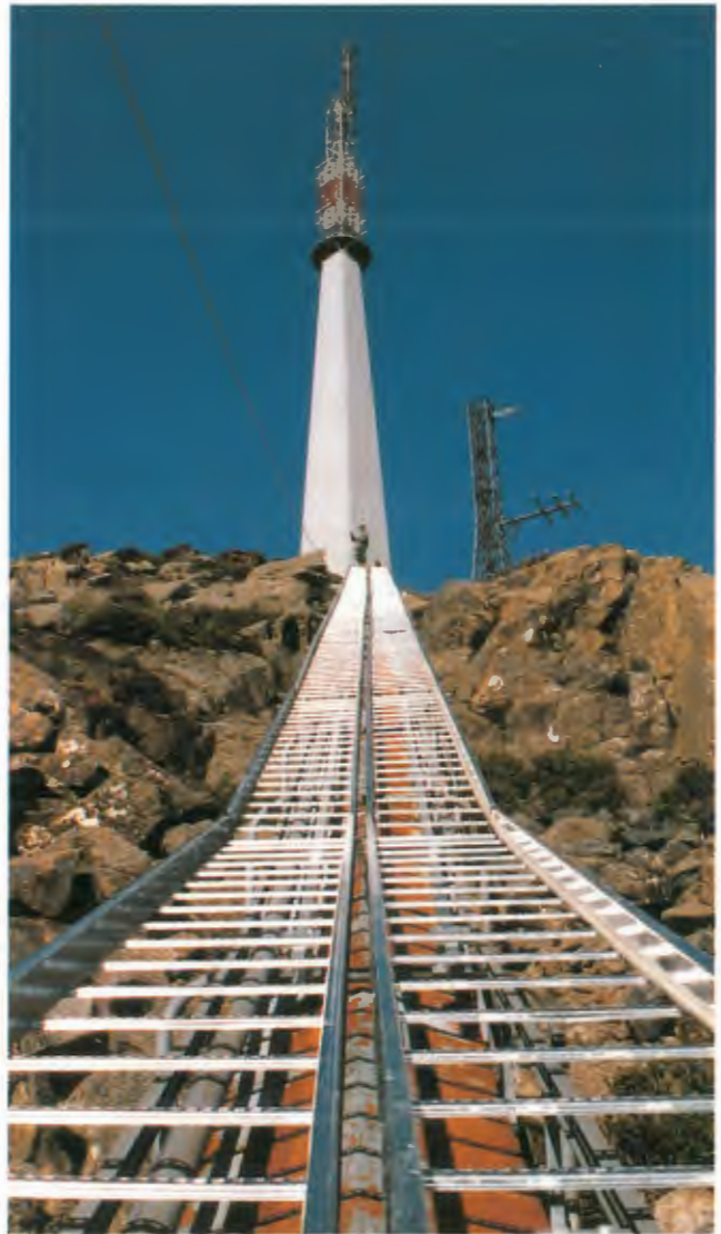
Radome removed and new cable gantry installed.
