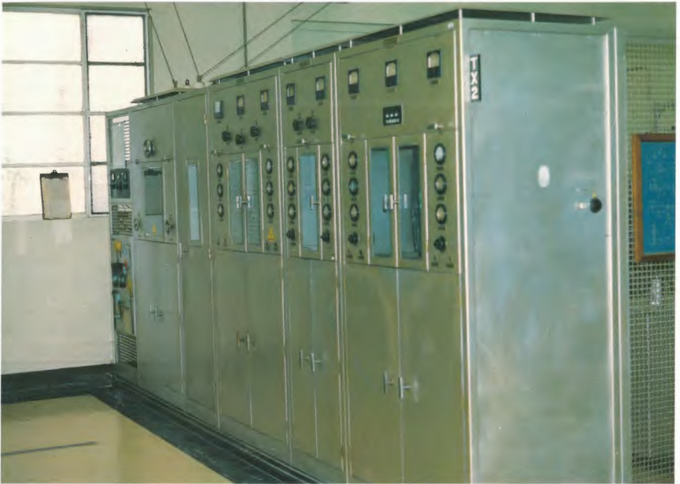
STC 10 kW type A880A transmitter installed VLQ 1943.
