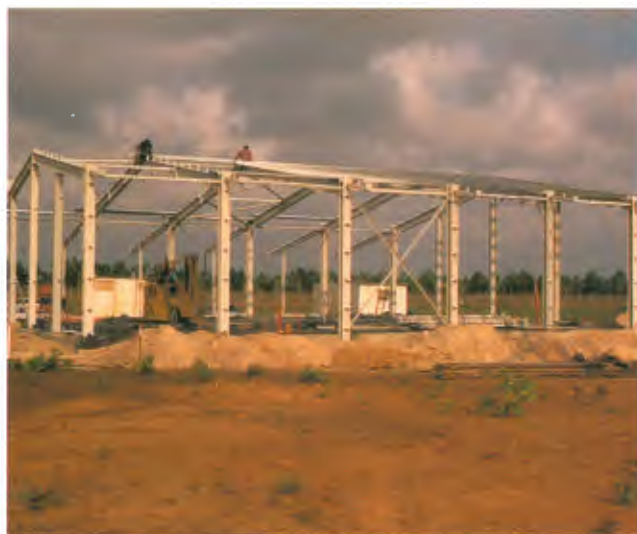
Building in early construction stage.
