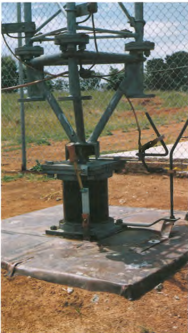
New mast base.
