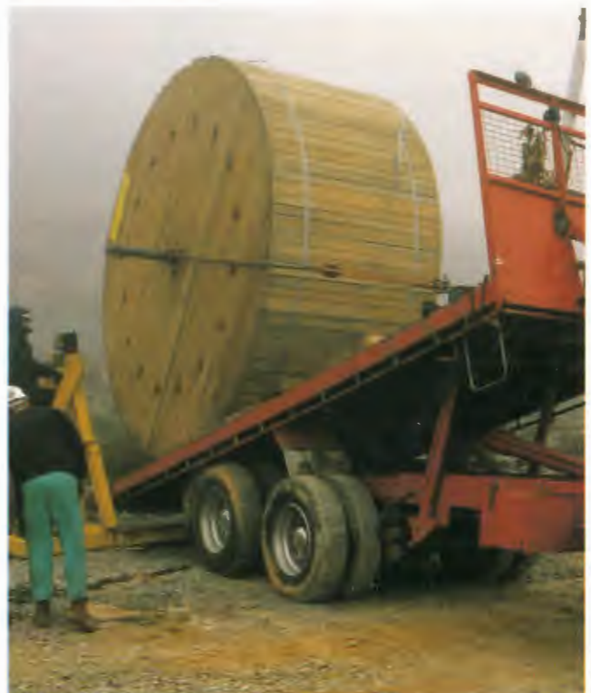
UHF feeder drum being placed on jacks.
