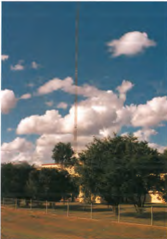
4QS station building hidden amongst the trees with radiator in background.
