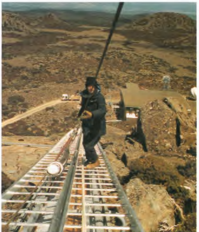
Installing the first 5 inch UHF feeder.
