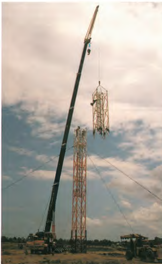
Mast construction in progress.
