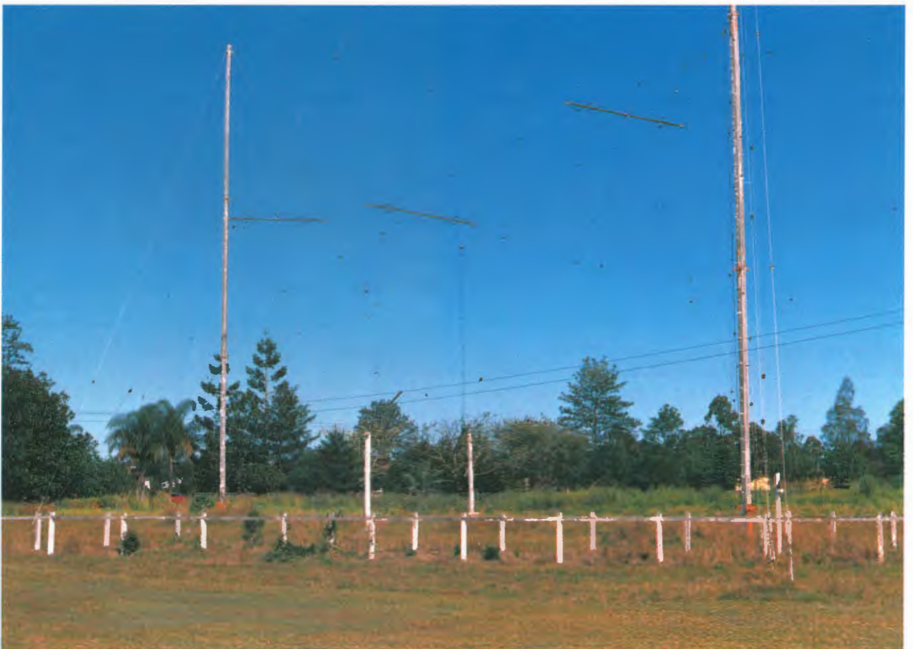
Part of early short wave aerial system at Bald Hills employing Oregon support masts.
