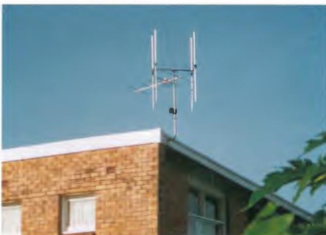
Horizontally polarised VHF Yagi and vertically polarised VHF phased array.
