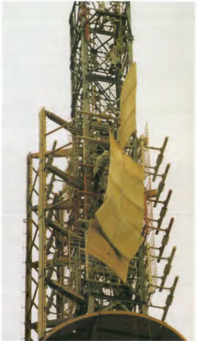
Removing last of the radome panels.
