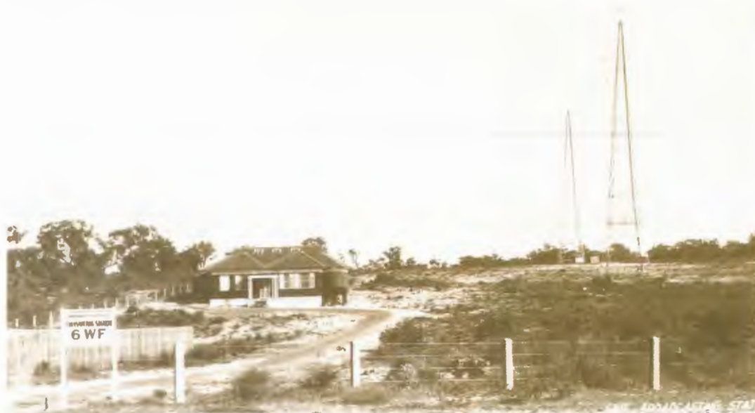
Transmitter building and aerial system as commissioned 1932.
