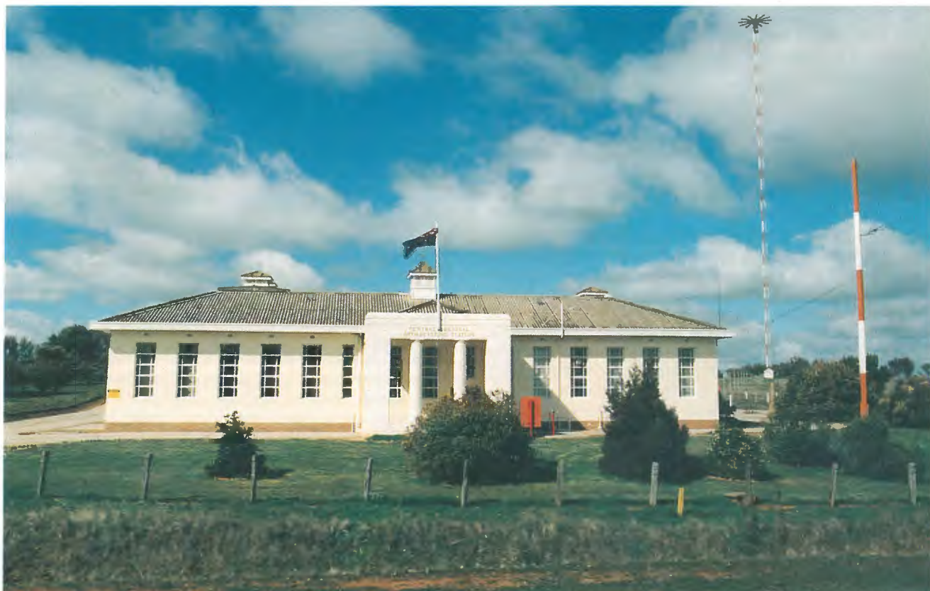
The magnificent building, typical of 10kW station designs in the late 1930's.
