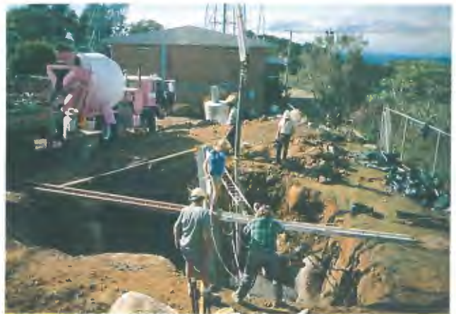
Pouring concrete into one of the tower footings.
