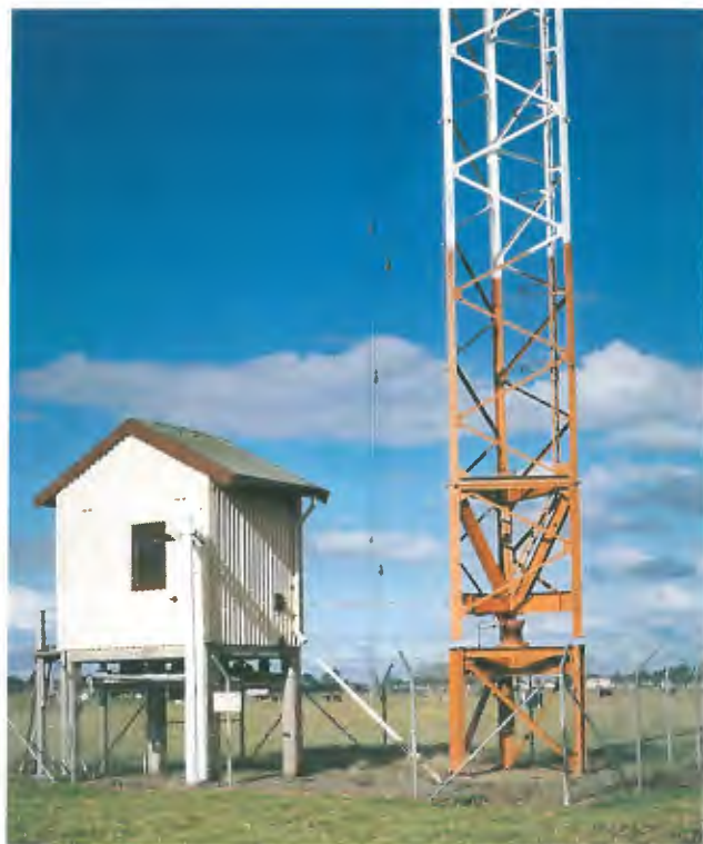
Elevated coupling hut and radiator base insulator.
