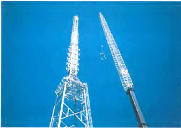
Crane hoisting material for antenna erection.
