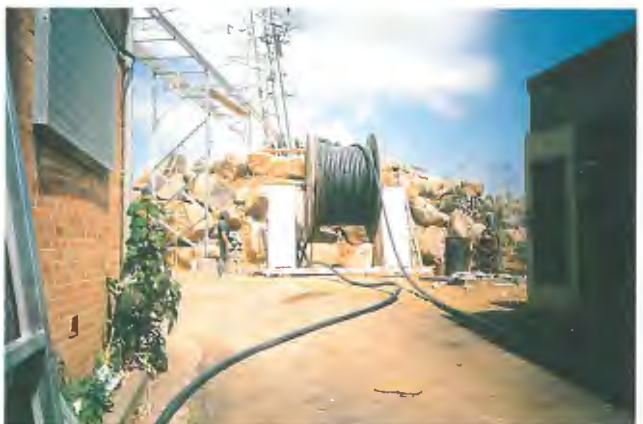
Coaxial feeder being set up.
