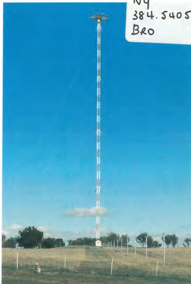
The 198m armature loaded radiator, operational since 1937.
