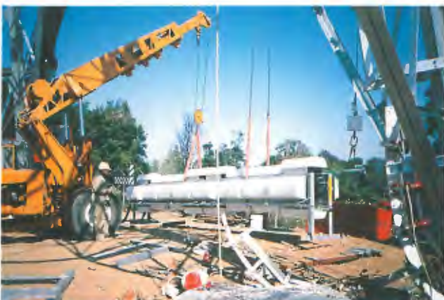
Antenna being prepared for hoisting.
