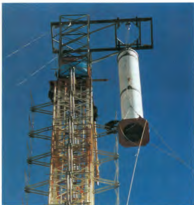
Lifting to Top of Tower with Travelling Gantry.
