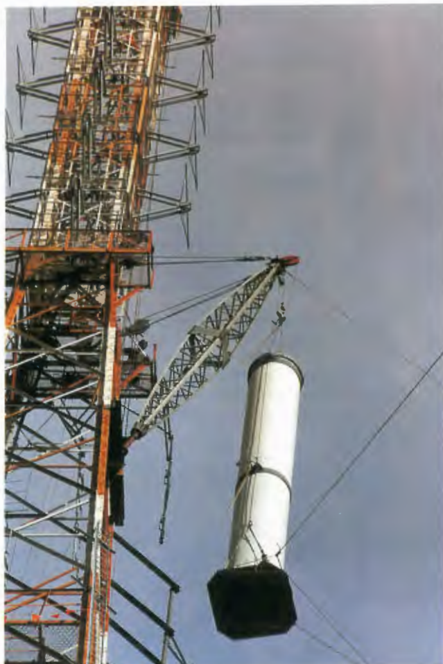
Lifting to 100 m Level with Side Mounted Jib Crane.
