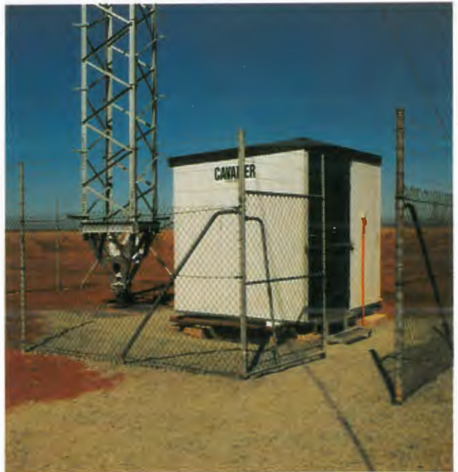
Mast Enclosure and ACU Building.
