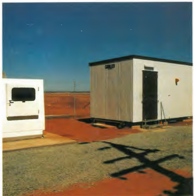
Diesel Building (L) and Transmitter Building.
