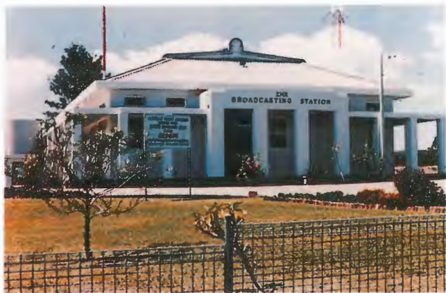
2NR transmitter building.
