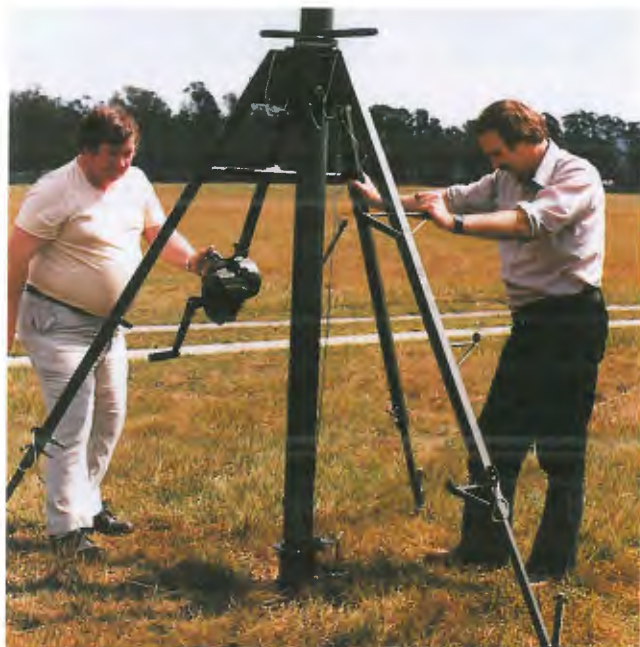
Lowering mast onto base insulator. Norm Pearce TA2(L) and Bob Heggarty STO1
