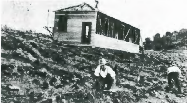
Building erection and earth mat installation Radio Hill 1926
