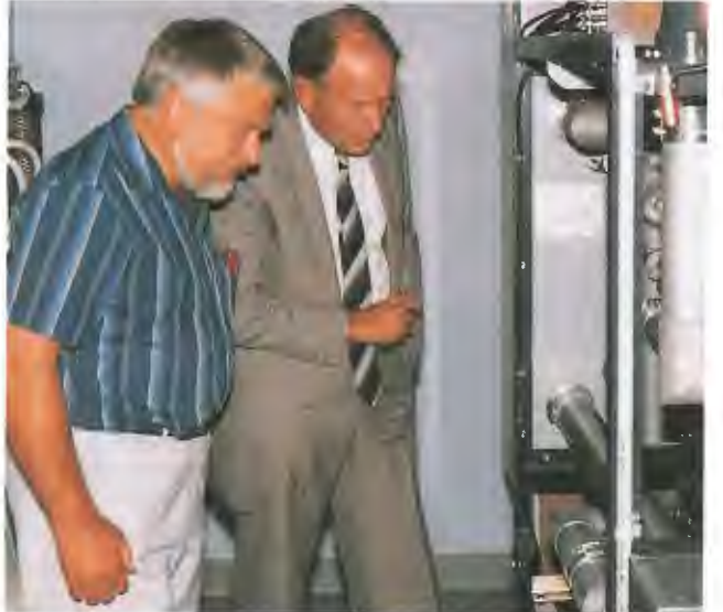
Don Benck (L) OIC Bickley and Mr Sebire inspecting SBS installation.
