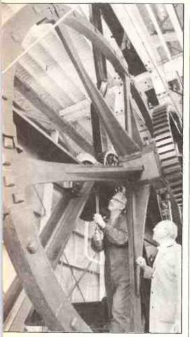
The flywheel of the Boulton and Watt steam engine.
