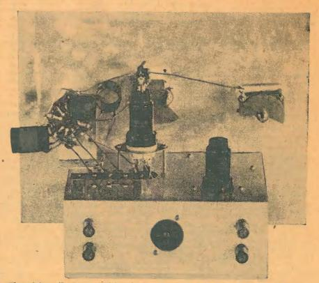
The set from the rear. Aerial and earth terminals at left, headphone terminals at right. All but the earth terminal are insulated from the chassis. Battery socket in the centre.
