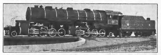
The largest locomotive ever shipped from the United States of America. This mighty engine was built by the American Locomotive Company at Schenectady, for the Pekin-Suivuan Railwayone of China's most important lines-constructed and operated entirely by Chinese. Locomotive and tender are 95 feet long, weigh 320 tons, and develop 3,000 horsepower. When in service it will be the largest in the world outside of the United States of America.
