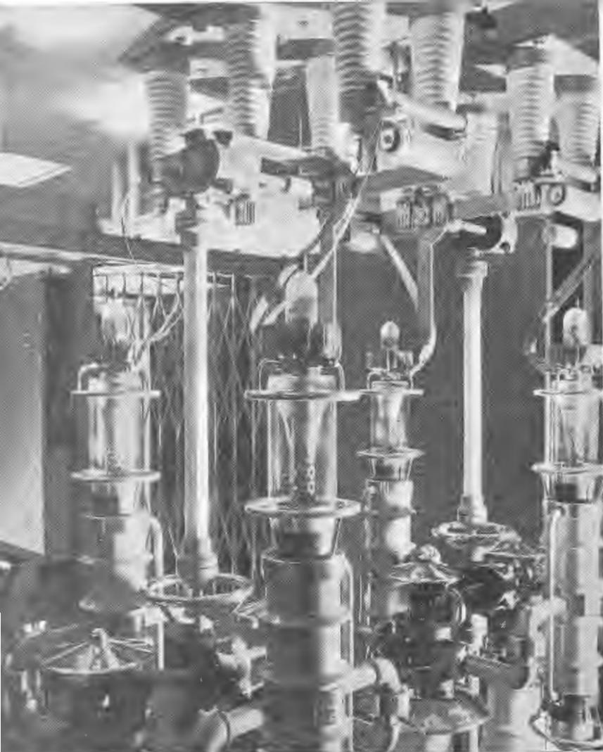
A 15,000 volt DC rectifier unit for use with the 100 kw. transmitter showing mercury vapour rectifier valves.
