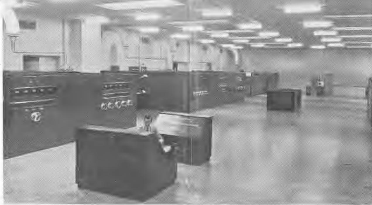
A view of the transmitter hall, showing the two 100 kw. transmitters in the foreground and the 50 kw. unit at the rear.
