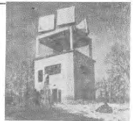
One of the seven microwave relay stations. A pair of shielded lens antennas provides two way transmission at 4000 Mc.
