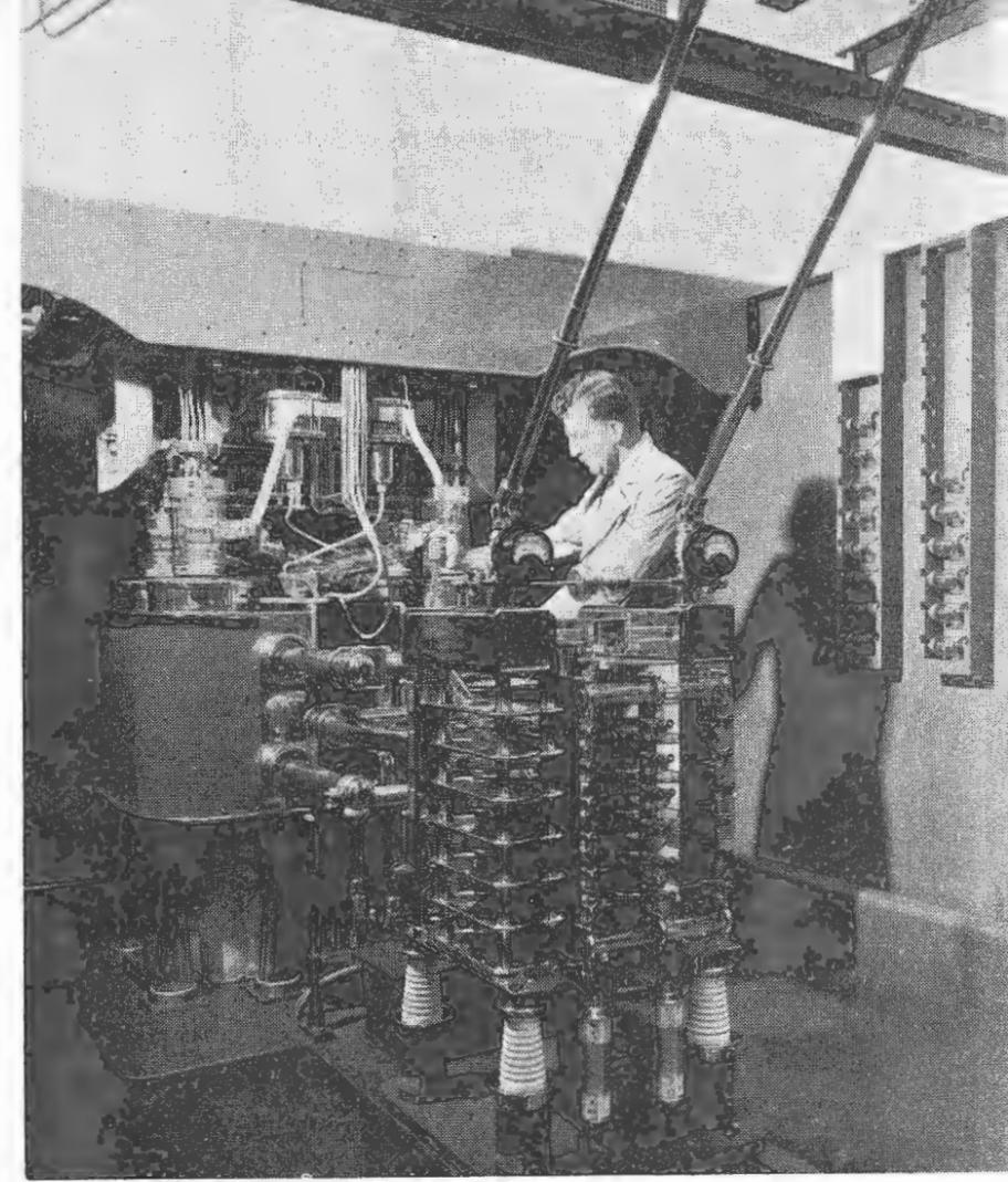
The Australian designed 100 kw. r-f power amplifier installed at Shepparton.
