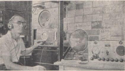
Dxer R. Simpson, of Sydney, winner of the second "Radio World" Shortwave Contest, at the controls of his home-built 10-valve Silver Marshall receiver. On the right is Mr. Simpson's version of the 13-valve Radiotron senior communications receiver, while in the centre is the Replogle combination world globe and time converter donated by the "Radio World" as first prize in the contest.
