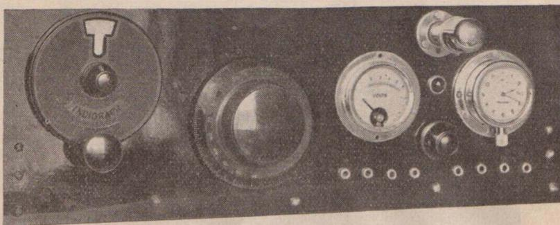
Complete with every gadget, including a clock, a filament voltmeter, and a dash light, which allows both to be easily read, this experimenter's s.w. set presents an imposing appearance.
