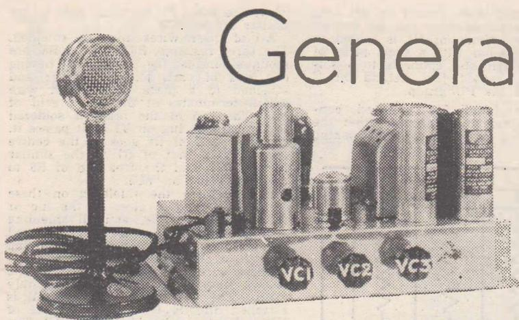
This photograph shows the complete assembly with a crystal type microphone standing alongside the amplifier.
