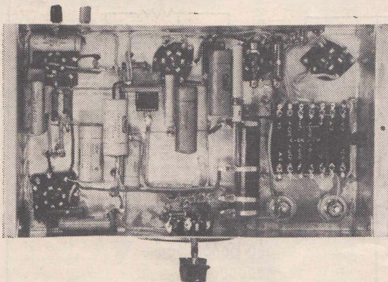
Another picture of the receiver showing the placement and wiring of parts below the chassis.
