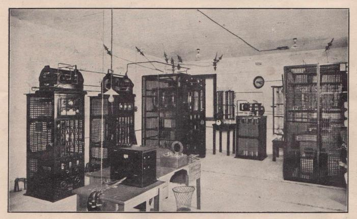
In case you don't know, th's is nt little Willie's Crystal Outfit --- it's Victoria's new Broadcasting Station 3LO. From left to right can be seen, the Master oscillator panel, modulator panel, 6KW amplifier, tuning gear and high voltage supply panel, containing the transformers, rectifier valves and smoother.
