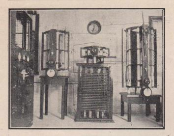
The Tuning Gear and closed circuit condenser at 3LO. The aerial lead-in can be seen at the top centre, the 6KW Amplifier panel being on the left.
