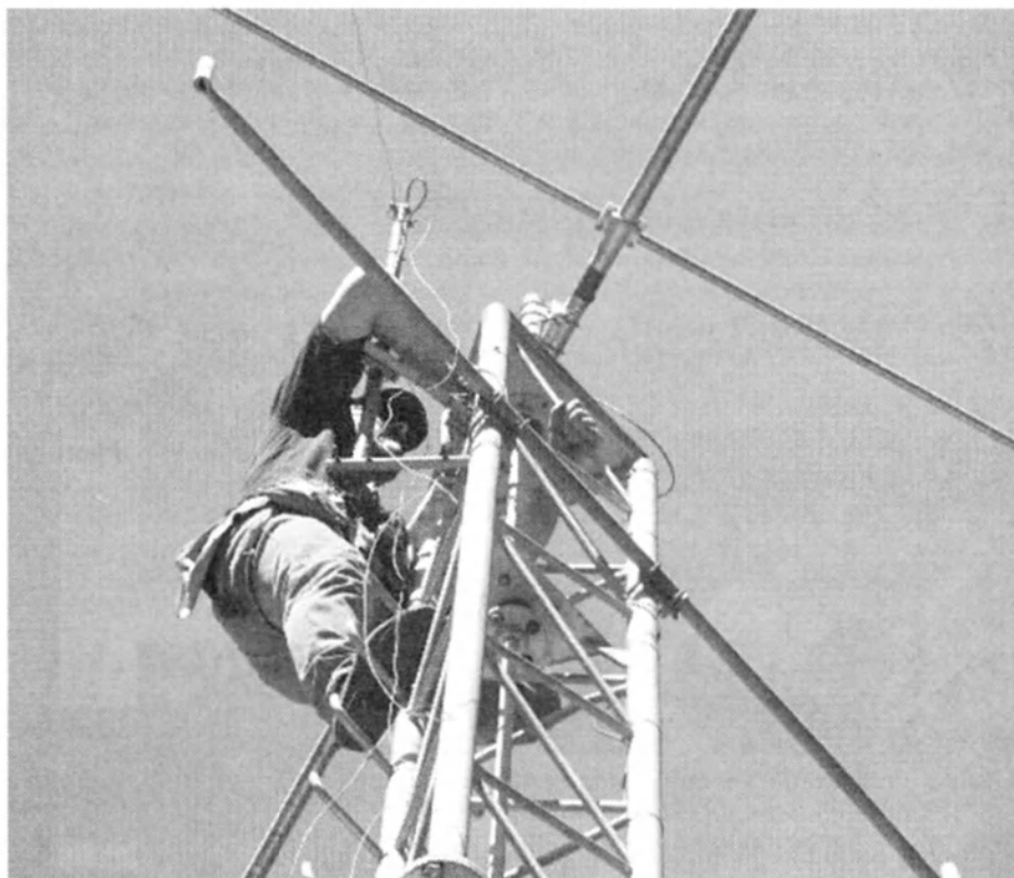
Photo 1. Mike Norris (Ulverstone Scout Leader) repairing the 40 m antenna
