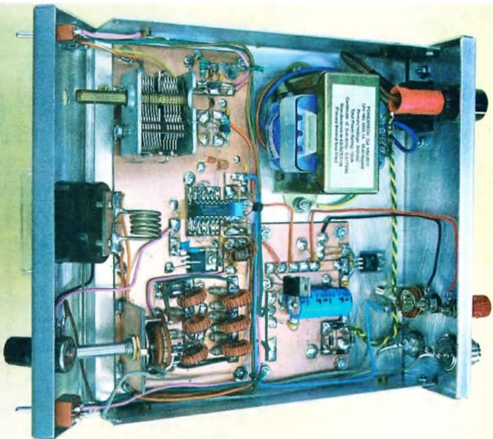
Photo 2 - Circuit board layouts (front panel lowered for clarity).
