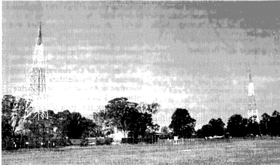
Figure 1: the NDB at Canberra Airport, one of many similar beacons scattered around Australia
