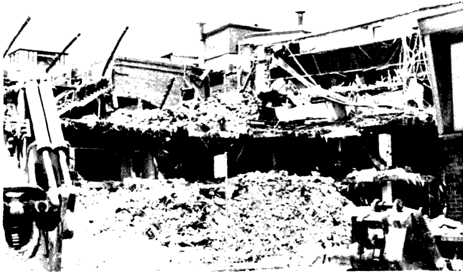
Newcastle Workers Club
