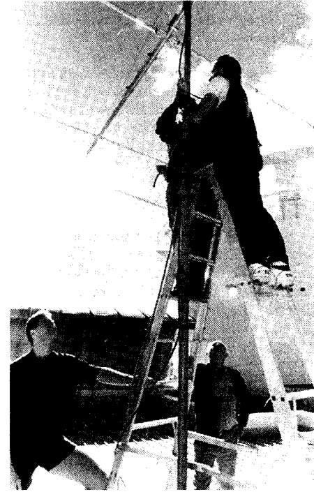
Erecting the TH6 antenna on the roof of Questacon / National Science and Technology Centre. On the ladder, John VK1ZX, George Briskey NSTC. Lower left Michael Goiser NSTC, Ted VK1AOP.
