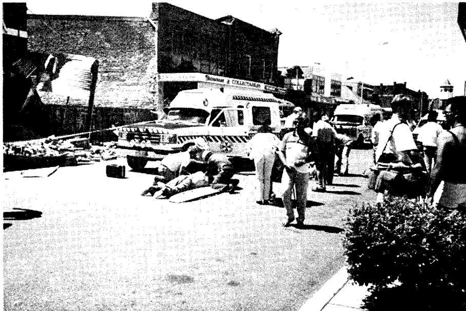
Beaumont Street Hamilton. First aid just after the earthquake.
