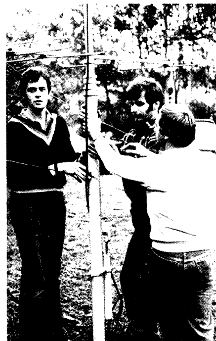
Albert VK3BQO, Ben VK3KLM and Peter VK3YZP working on the 13 metre, pump-up mast at Camp Jungai.
