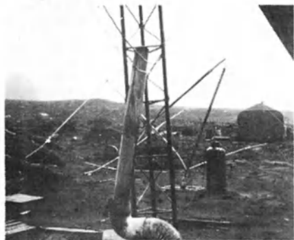
Bent and twisted antennas after strong winds.
