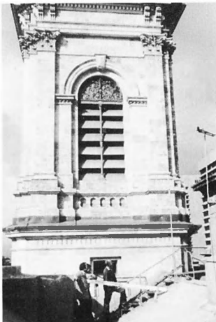
Trap vertical on roof of GPO. Maurie VK5ZU (right) and Dave Hogben of Australia Post.
