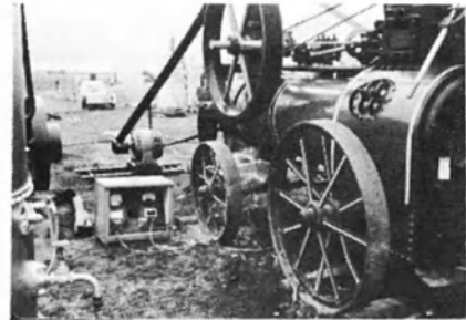
Generator and Steam Engine
