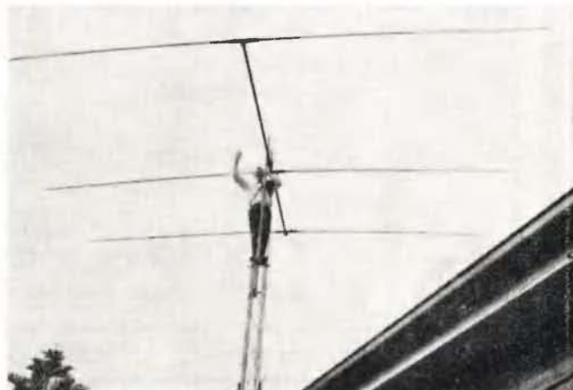
Beam 30 feet up on not yet cranked up steel mast. Junior op. on mast.
