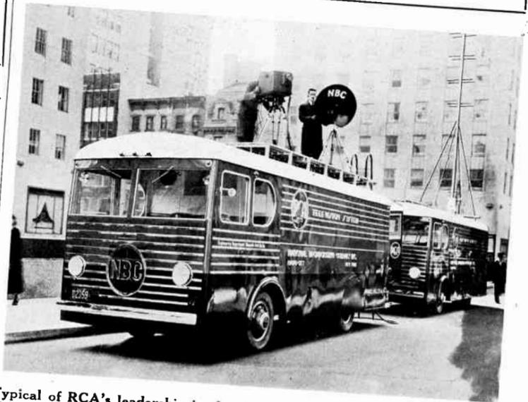
Typical of RCA's leadership in the development of television is this television transmitter caravan which will be used in New York in 1938. Note the iconoscope camera and antenna on the roofs of the cars. This equipment will transmit by ultra-short wave to the Empire State Building atop which is the main transmitter used in RCA's television broadcasts
