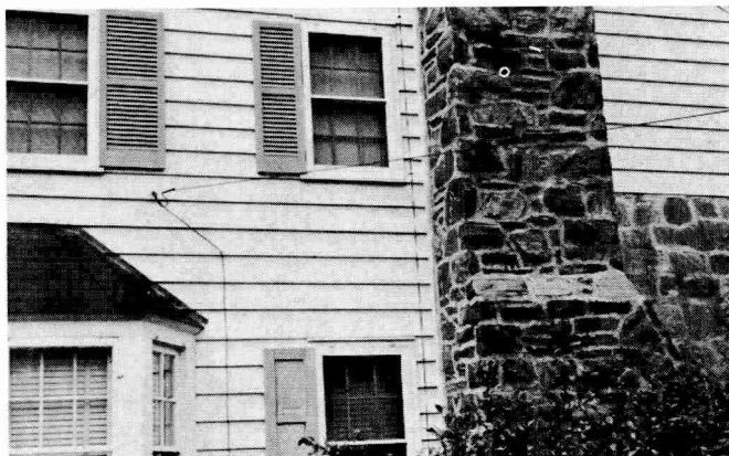
The transmission line should follow a direct route, and it should be spaced at least six inches from power and telephone lines.
