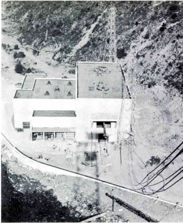
Jim Creek transmitter building (Official U. S. Navy Photos)
