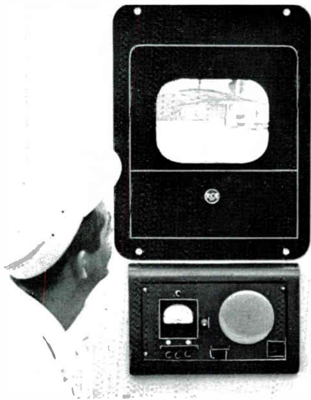
Powerhouse control operator checks plant's gate
