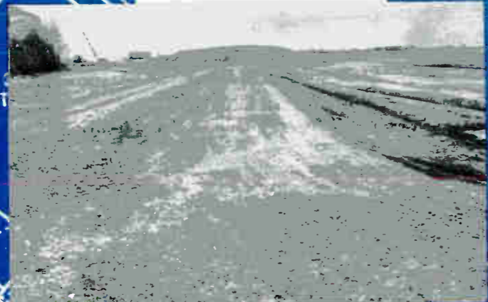
And the earth is pushed until it is molded into the proper shape for the entrance
