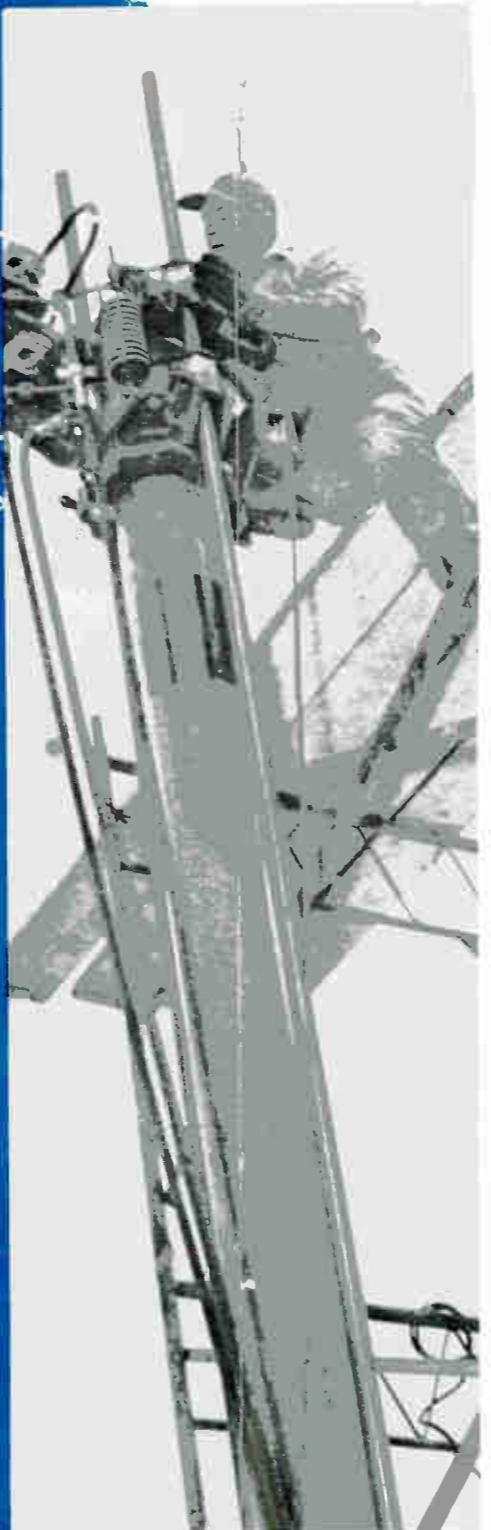
Adjustment is made to the jack which is to lift the pre-poured building floors into position
