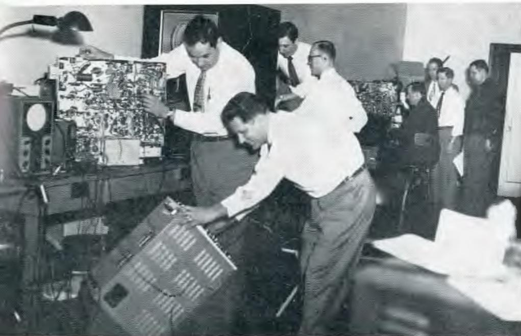
BEHIND SCENES at Astoria (L. I.) color labs. Howard Spencer & Joe Fissmer (l. to r., foreground) check receiver color balance with cathode-ray oscilloscope
