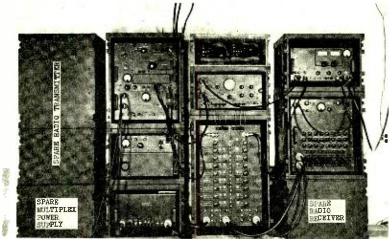
Fig. 2—The AN/TRC-5 equipment developed for the U. S. Army Signal Corps.
