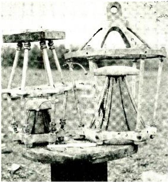
Fig. 21—Two types of insulators used in guy wires of WJZ antenna.
