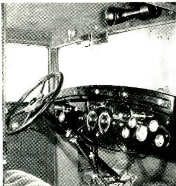
Fig. 1—Early two-dial receiver. Custom installation.
