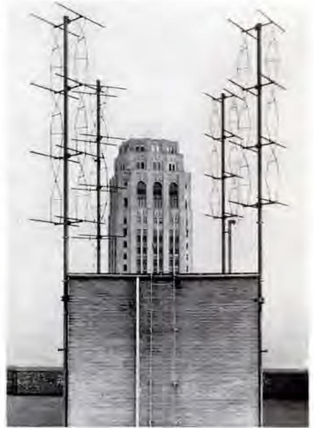
Modernistic "Trees" bear crop of words for Europe—Central office of RCA Communications is in downtown New York. Its transmitters in the open country were formerly connected with New York only by wire. Now RCA engineers send ultra-high frequency waves from these odd-looking antennas. The waves automatically operate RCA's transatlantic transmitters at New Brunswick, N. J. Result is improved service.
