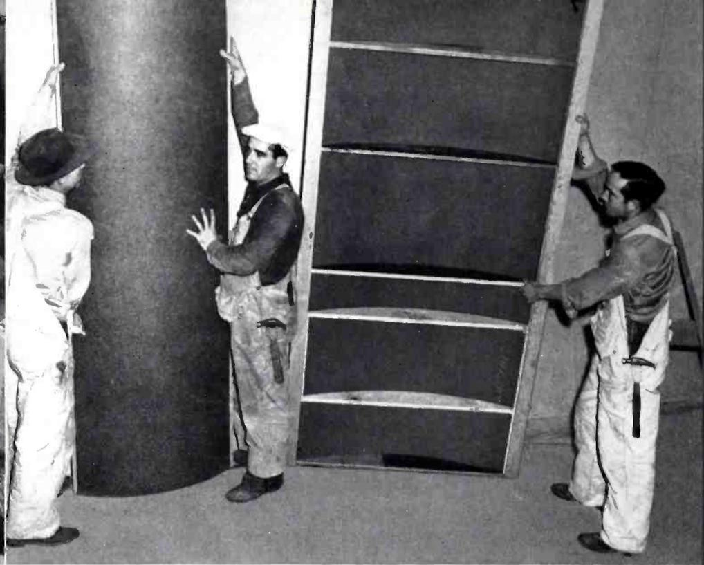
**FIG. 4.** (Left, Above) The KRON ceilings are supported at their edges by the isolated walls, and by felt isolators attached to the concrete slab above. Ventilating ducts are similarly supported by felt isolators.
