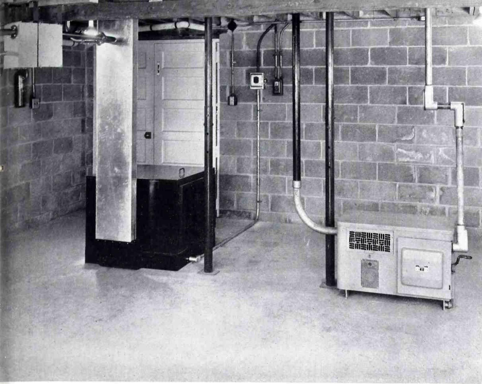
FIG. 5. (at left) A view, of the basement directly under the BTF-10B transmitter, showing the blower, plate transformer, harmonic filter, and transmission line monitor. Note that a special duct is used to carry the air from the blower through the transmitter base to the power amplifiers.
