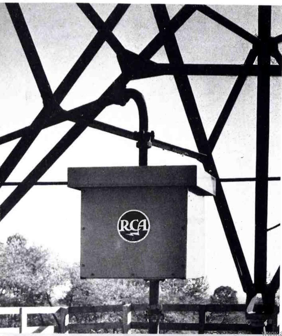
and also supports the FM antenna (an RCA BF--3B Superturnstile, 3 bay). Isolation is provided by the RCA BAF-4A AM/FM Isolation Unit shown in Figure 6. Duplicate transmission lines are provided for each tower and we used Communication Products Co. Seal-o-Flange,  $\frac{7}{8}$ " 51-ohm line for AM and  $1\frac{5}{8}$ " 51-ohm line for FM.
