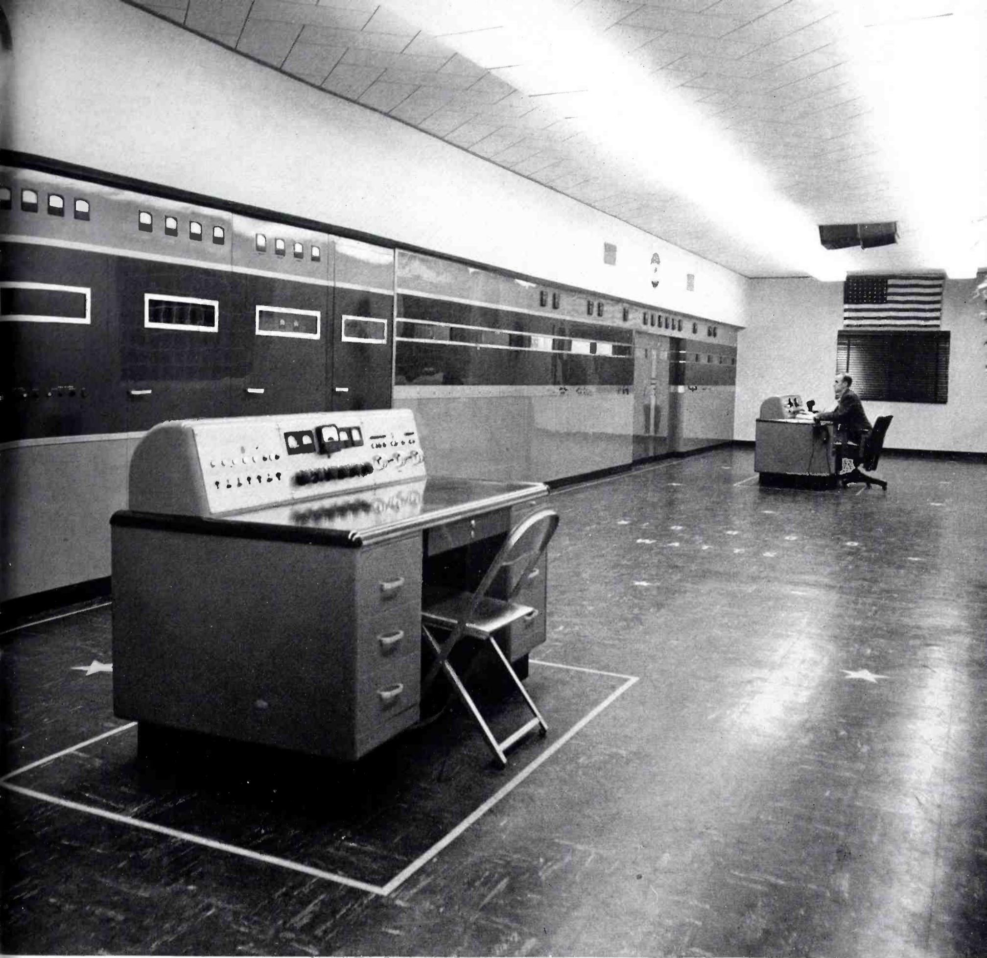
**FIG. 24.** *The interior of the "Station of the Stars" is no less beautiful, at least to the eyes of an engineer. Nearly 80 feet of unbroken transmitter front—and all of it the newest and finest. In the left foreground is the RCA 10-E (10 KW standby) transmitter while at the further end is the new RCA 50-F 50 KW transmitter.*
