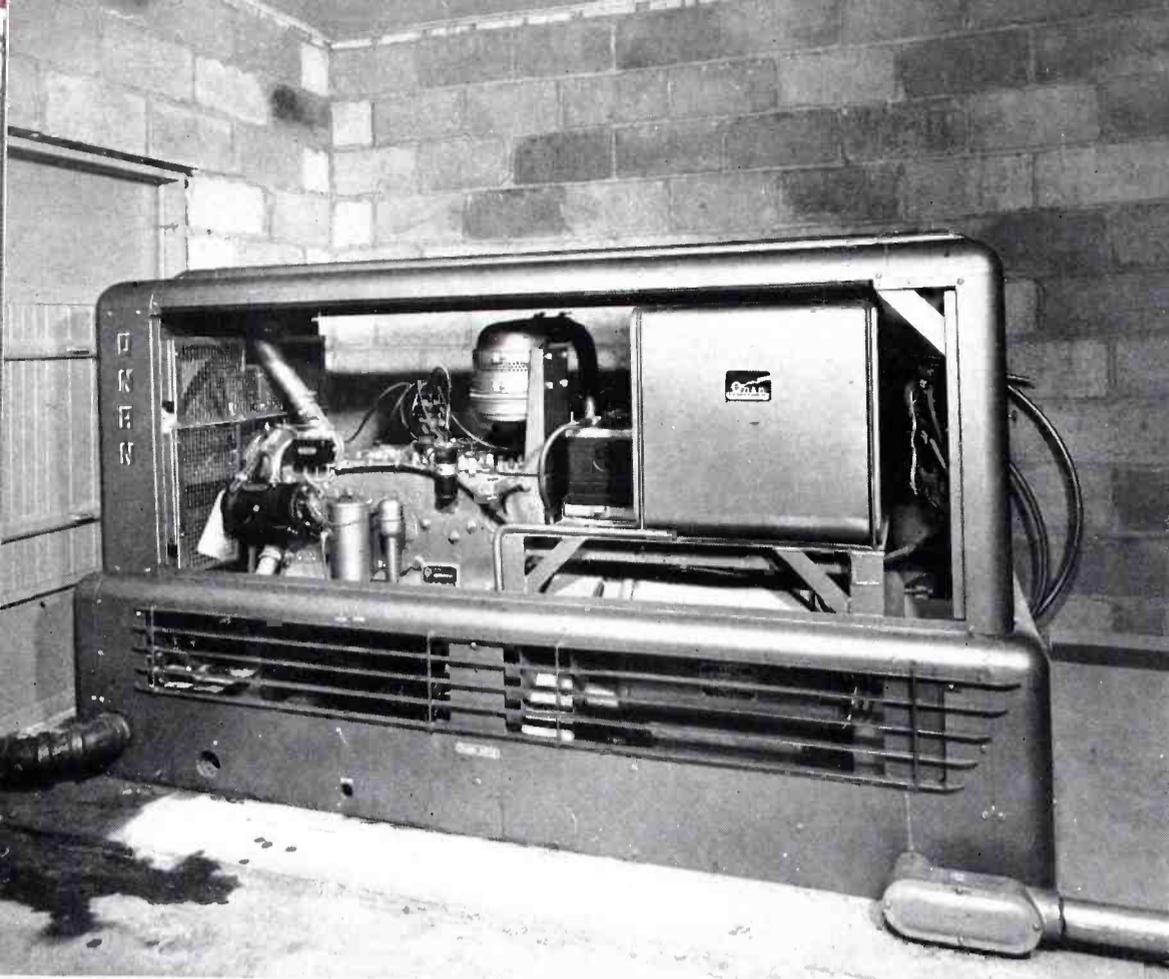
**FIG. 4.** (above) The standby power plant located in the WJPG-FM transmitter house consists of a six-cylinder gasoline driven Onan motor which develops 35,000 watts. It is equipped with undervoltage relays which automatically start the generator and switch the load from the power line to the generator in the event of transmission line failure.
