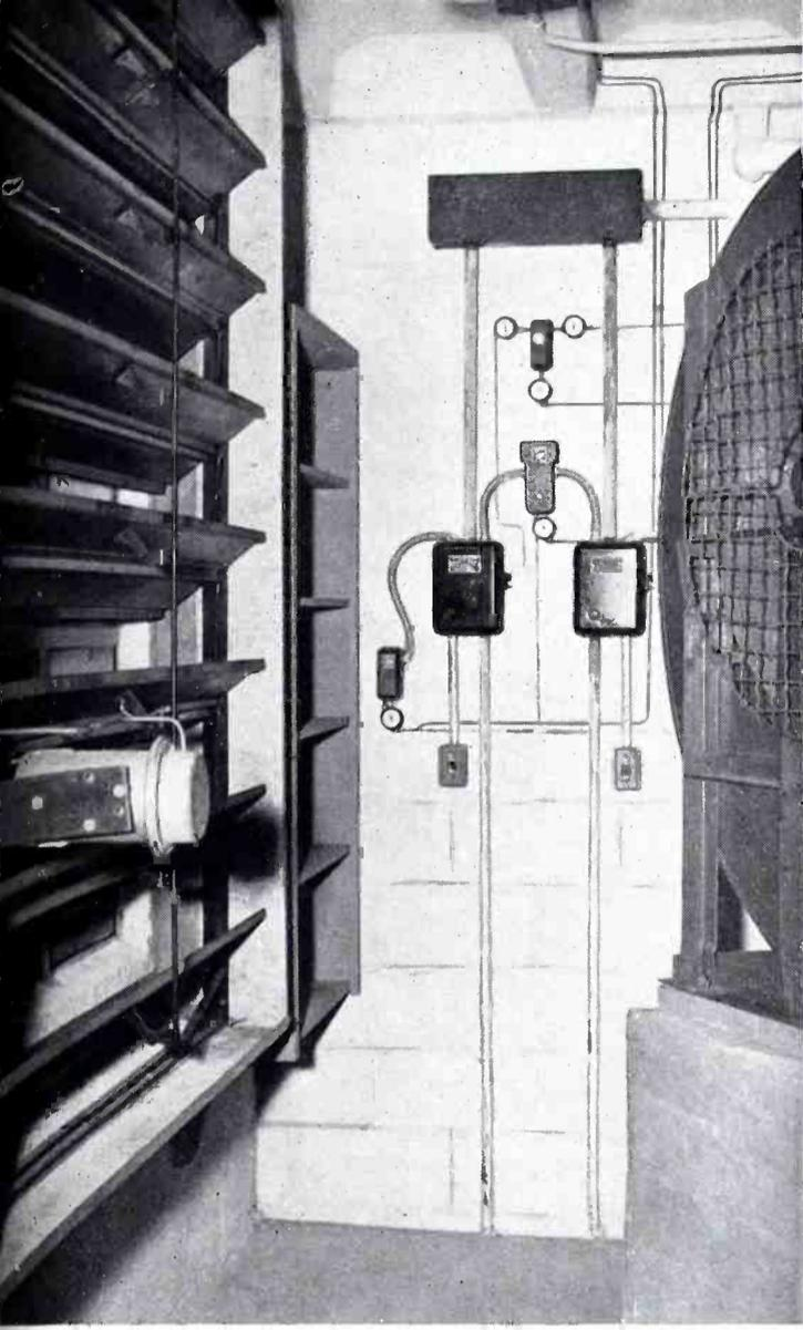
**FIG. 10.** A corner of the blower room. One of the blowers may be seen at the right. At the left are the thermostatically-controlled inlet dampers. Blower controls are on the back wall.
