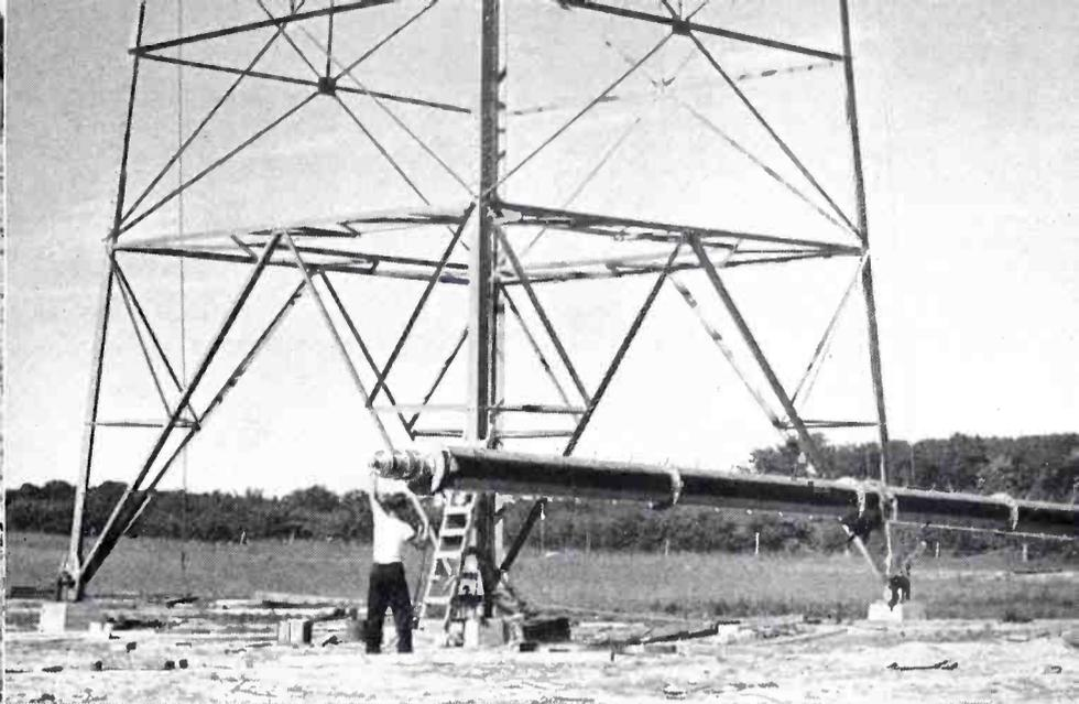
**FIG. 8.** (above) *Completely assembled (with polyethylene sheets covering the full length slots and with beacon attached) the Pylon is ready to start its way up the tower.*
