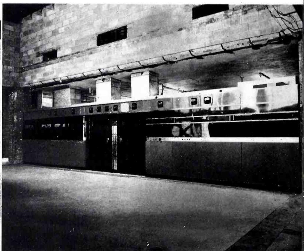
**FIG. 9.** This illustration shows the 50-F transmitter in place before the drop wall and wall finish were completed (see text). The outlet air ducts from the modulator, power amplifier, and r-f driver stages can be seen leading up from the transmitter proper into the room ceiling.
