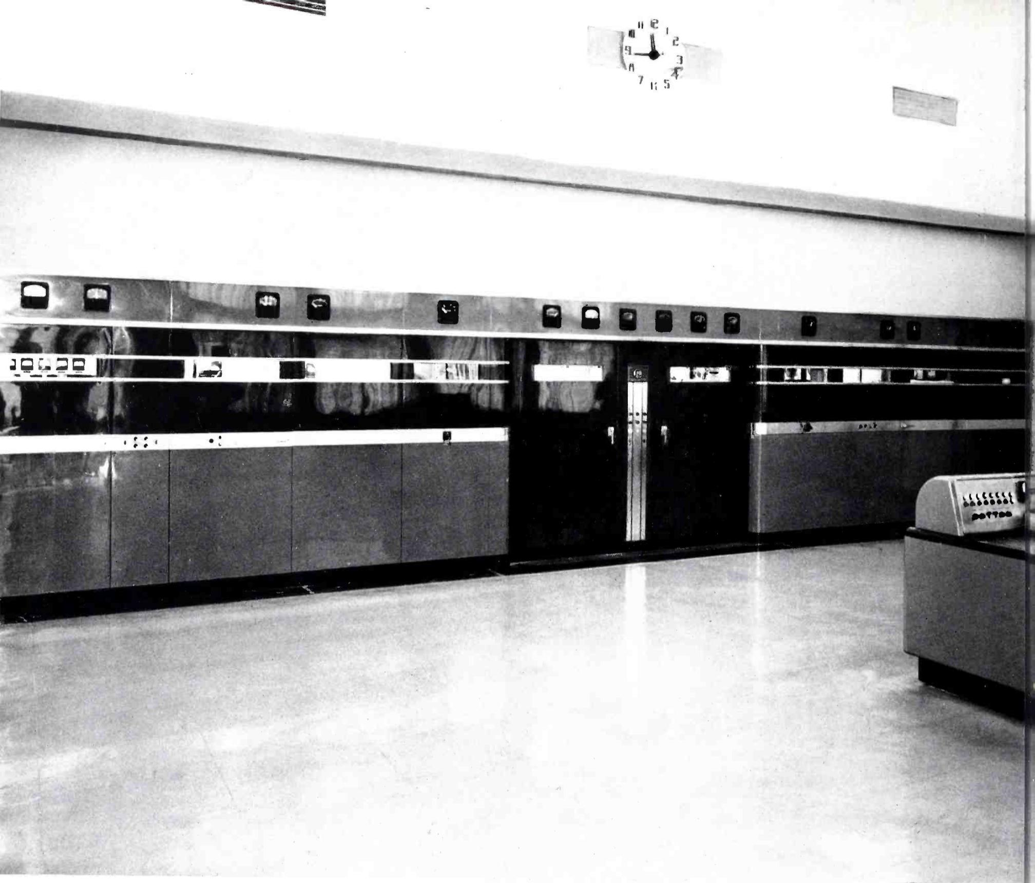
**FIG. 3.** *The WGAR transmitter room is rectangular in shape. The RCA Type BTA-50F 50 KW transmitter forms one of the long sides of the room while the other long side is of glass brick. The operating console is in the center of the room facing the 50 KW transmitter. Clock and ventilating louvres are located in the drop wall above the transmitter.*
