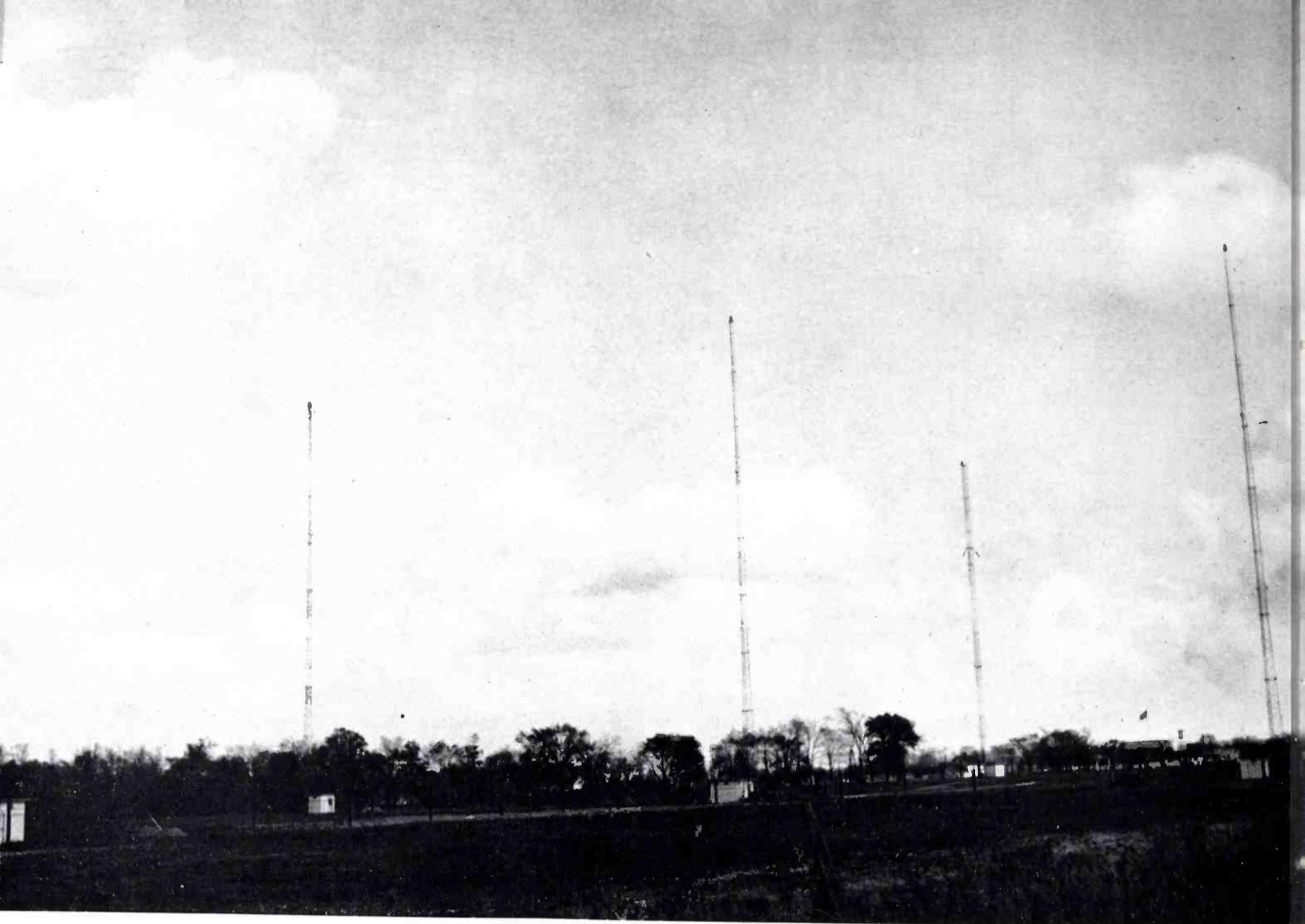
**FIG. 12.** *WGAR's 5-tower directional array is shown in this illustration. The four outer towers are arranged in a rhombic with the fifth tower at the approximate center, (see Fig. 14). The phasing and power dividing networks are located in the center tuning house which is the physical, as well as the electrical, center of the array.*
