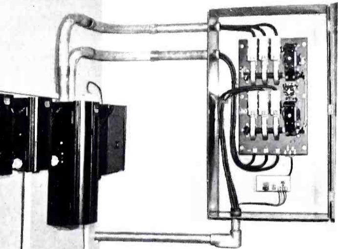
**FIG. 5.** (left) The various power switches in the WJPG-FM building are located as shown here. From left to right are the telephone termination cabinets and the power changeover switch for the Onan standby power plant.
