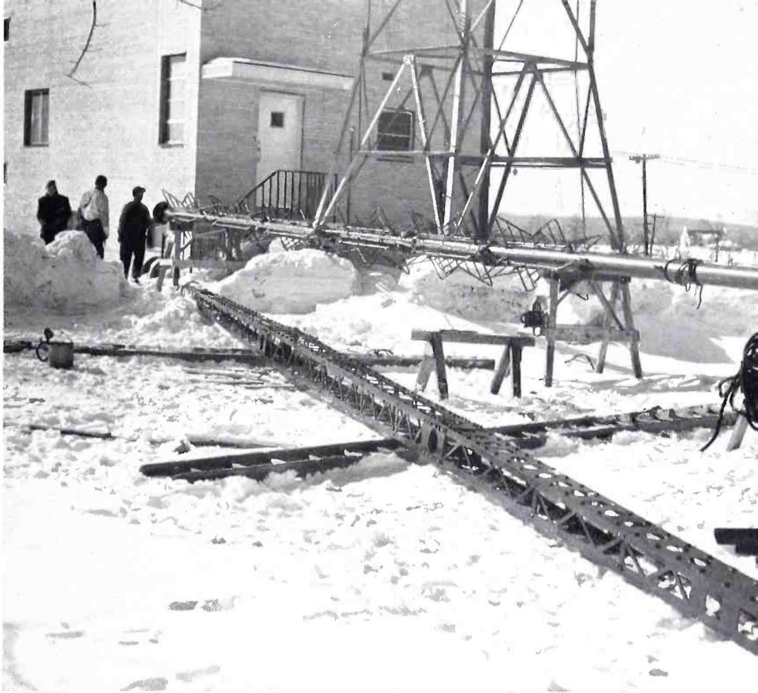
**FIG. 6.** (Above) A longer gin pole (see foreground) was used in raising the RCA 6-section TV superturnstile which is shown here.
