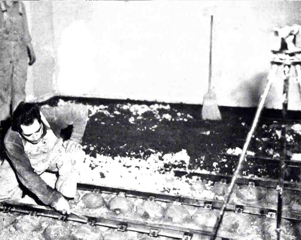
**FIG. 5.** (Right, Above) Polycylinders prefabricated from  $\frac{1}{8}$ " tempered masonite over randomly spaced ribs were scribed to fit the ceiling contour. Half-round moulding strips were milled to cover nailing strips. Where Polycylinders were joined, masonite was counter sunk and perforated paper tape and Egyptian cement were used to cover cracks.
