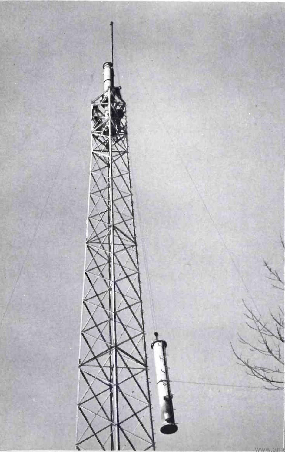
**FIG. 5.** (Below) *With the second Pylon section in position, riggers are securing thru-bolts to complete the FM Pylon installation.*
