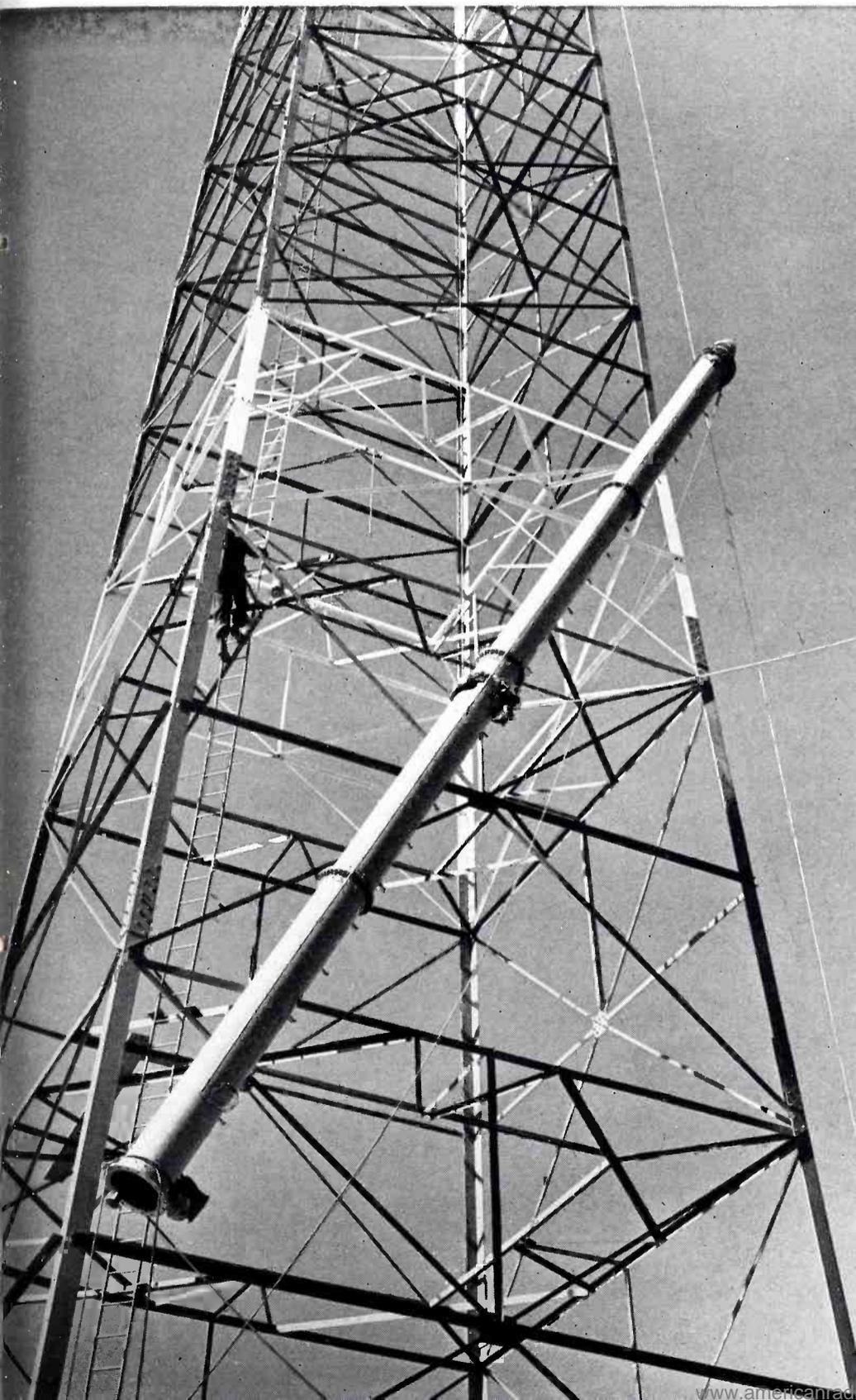
**FIG. 10.** (below) *With the Pylon nearly raised to full tower height, riggers are getting ready to mount the antenna atop the 325-foot structure.*
