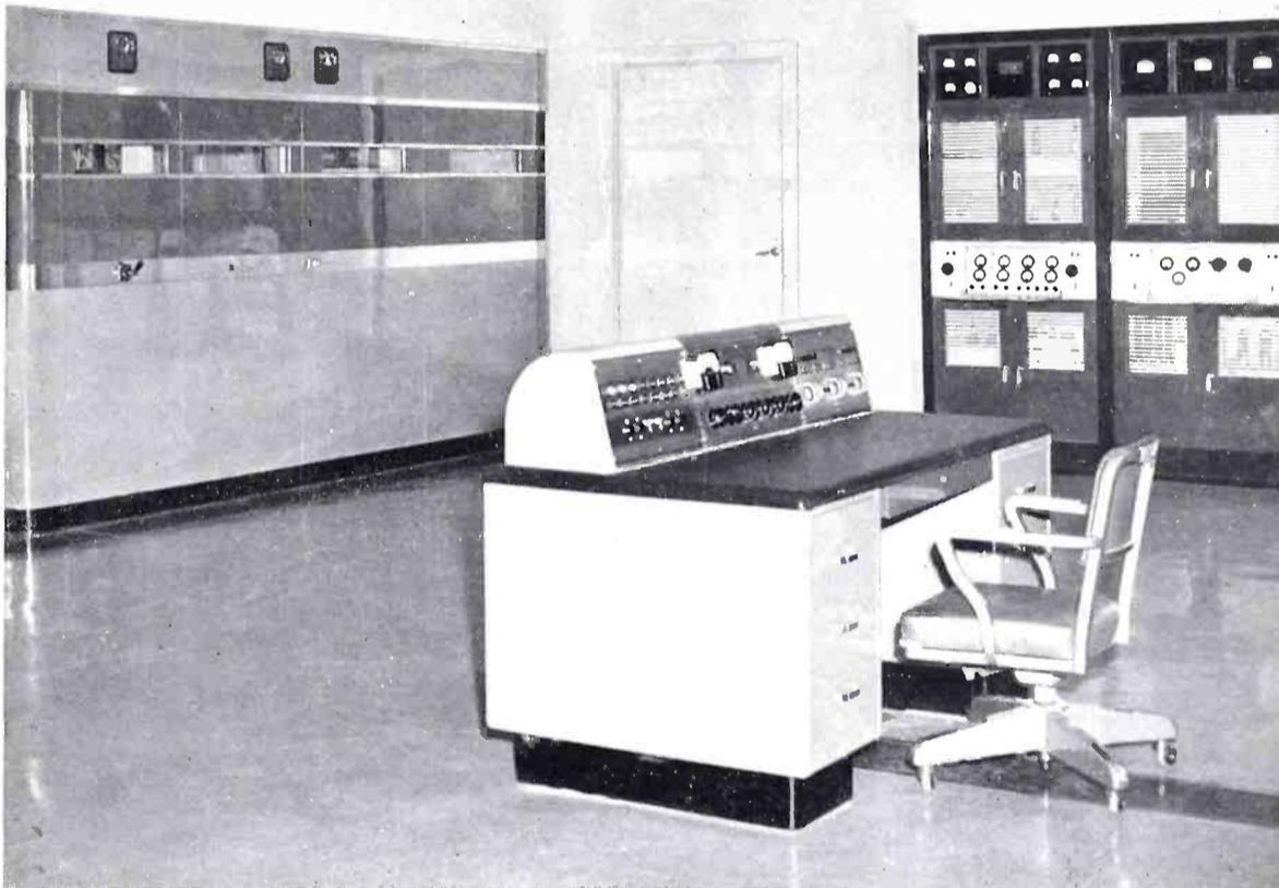
**FIG. 5.** (above) In the wall to the right of the operator's console is WGAR's old transmitter, an RCA 5-D which, in an emergency, can be operated from the station's 30 KVA deisel-generator.
