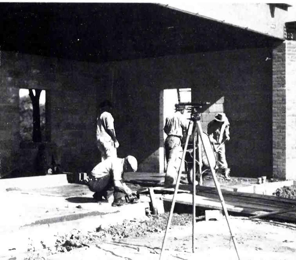
**FIG. 8.** This shows the 50 KW transmitter area after pouring of the floor. Set in the floor at the front of this area is the input air duct. The large round openings in the top of this duct are the air inlets to the several stages of the transmitter.
