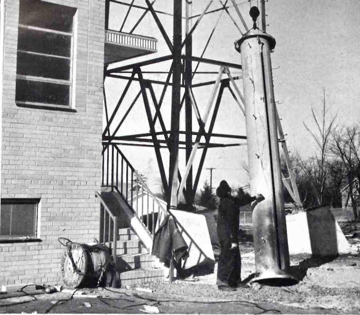
**FIG. 3.** (Above) *With cables attached for hoisting, the first Heavy-Duty Pylon section is ready to start its way up the tower.*
