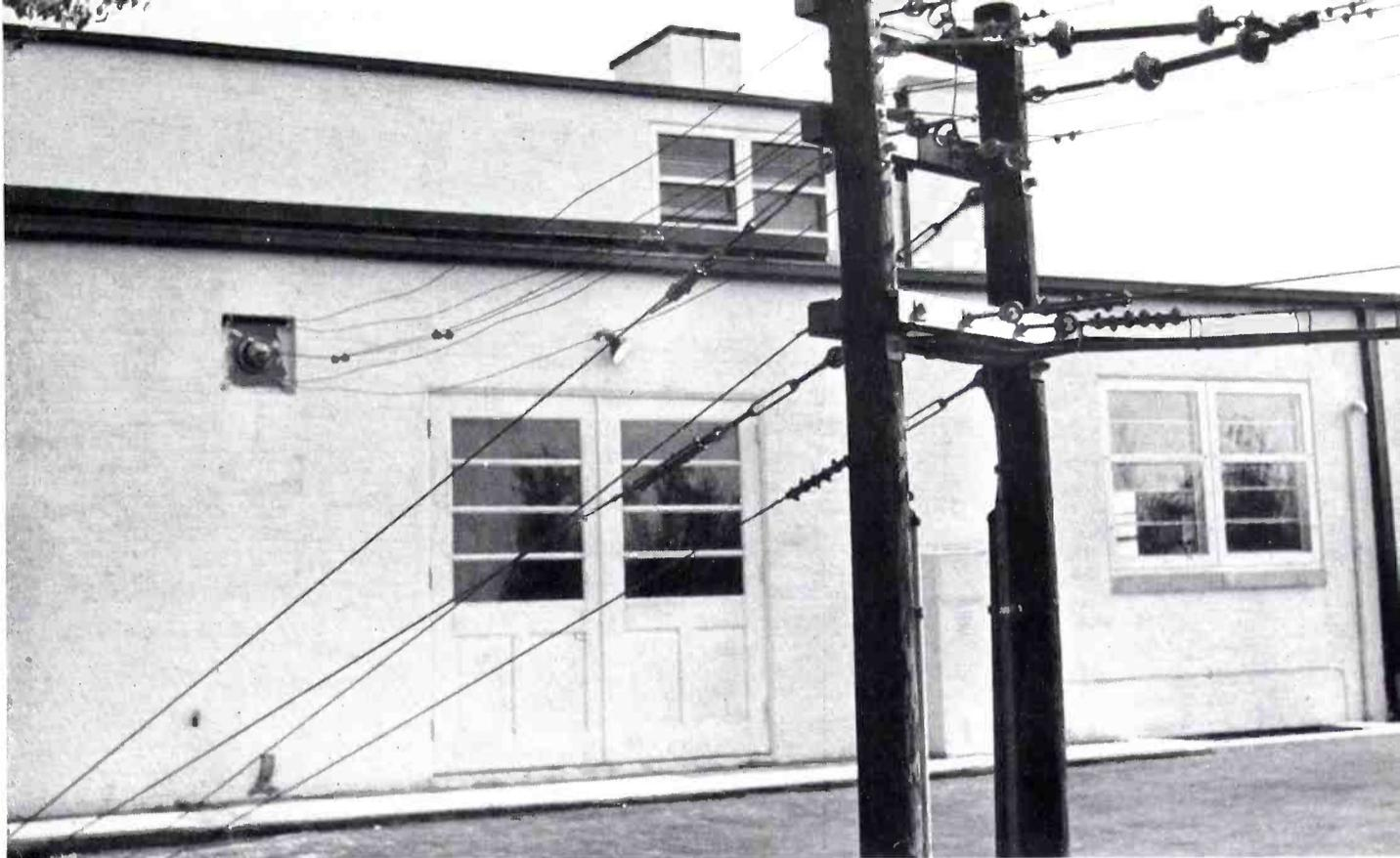
**FIG. 17.** (right) *Standard RCA 6-wire brackets were used to support the WGAR transmission lines at all points except the terminations. This view shows a part of the line installation before the towers were erected. Total length of lines employed is approximately 2800 feet.*
