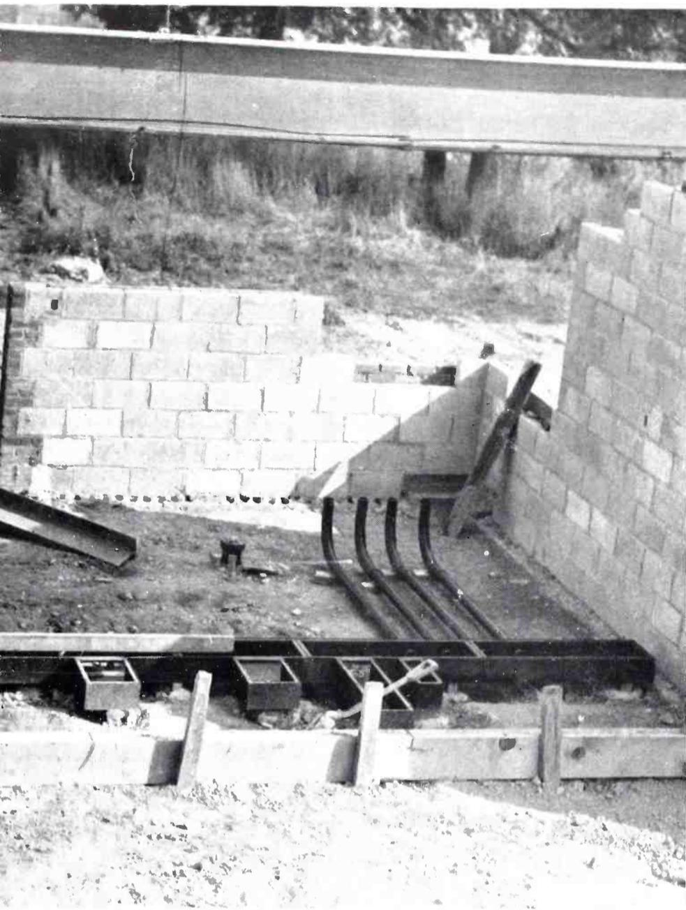
**FIG. 6.** Foundation walls for the WGAR building consist of concrete block, with air spaces of each course filled with concrete. Above ground walls are concrete block faced with brick painted white. This illustration shows the space for the 5-D transmitter, with the wiring trenches and conduit in place preparatory to pouring the concrete floor.
