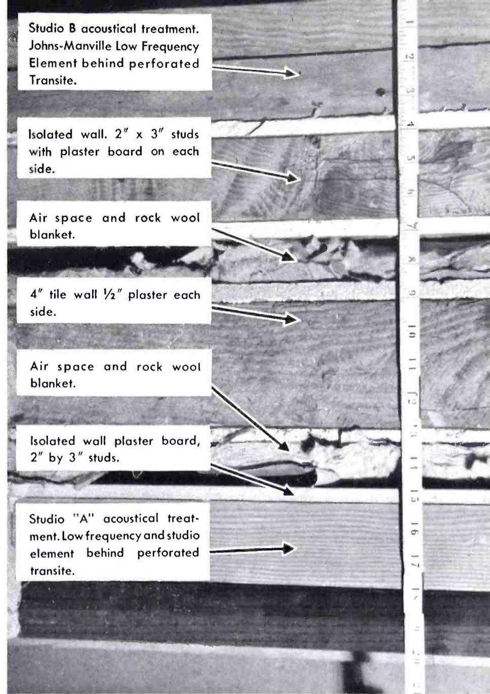
FIG. 2. (Above) Cross-sectional view illustrating the acoustical treatment employed in the construction of KRON's Sound Isolation Walls.
