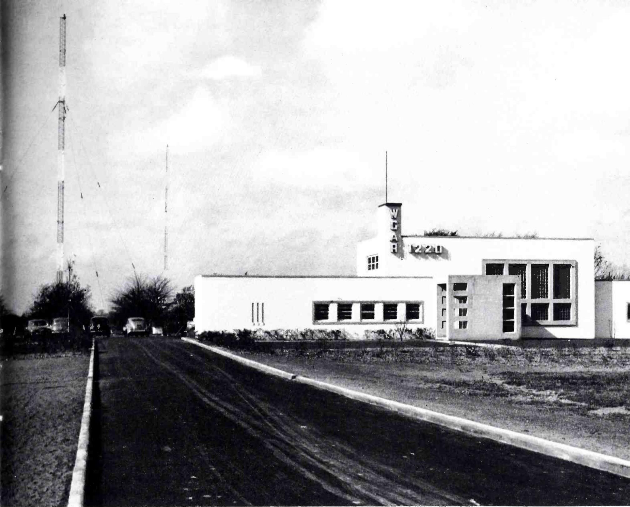
**FIG. 2.** *WGAR's new and modern plant is located thirteen miles south of Cleveland. Installed here is WGAR's new RCA 50 KW transmitter, the RCA 5 KW transmitter (for standby) and an RCA 3 KW FM transmitter.*
