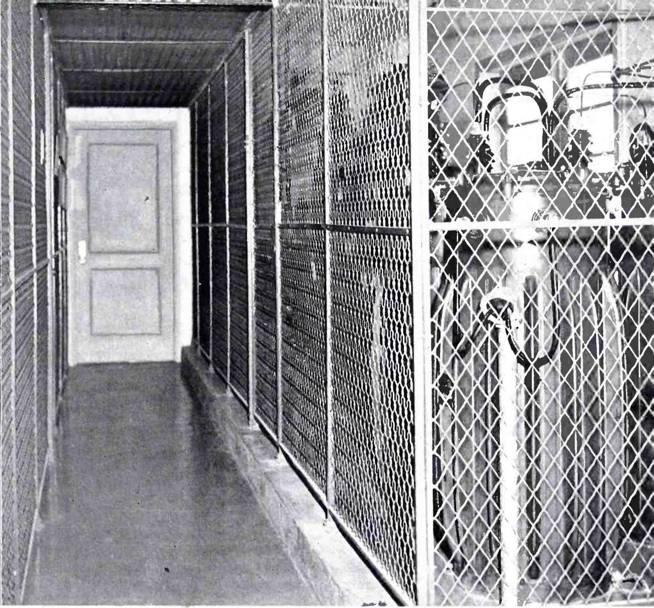
**FIG. 11.** Visitors can be taken through this protected aisle-way behind the 50 KW transmitter. At the left of the aisle is the transmitter proper. At the right, the transformer enclosure (note oil curb).
