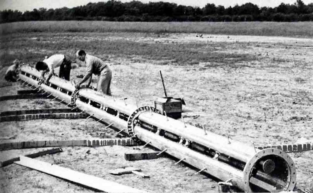
**FIG. 7.** (above) *All Pylon assembly work was done on the ground. The four sections were bolted together at the flanges, and transmission line harness was inserted prior to erection.*
