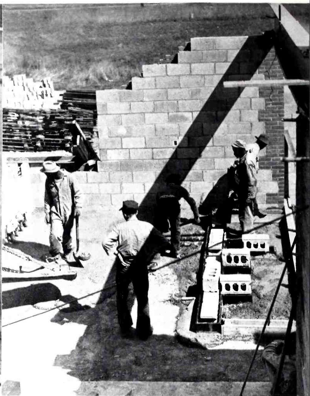
**FIG. 7.** This illustration shows the same area (as in Fig. 6) during the actual operation of pouring the floor. A part of the enclosure which forms the wall of the transmitter room may be seen at the right. Access to the area in back of the 5-D is provided by a door at the left of the transmitter (see Fig. 5).
