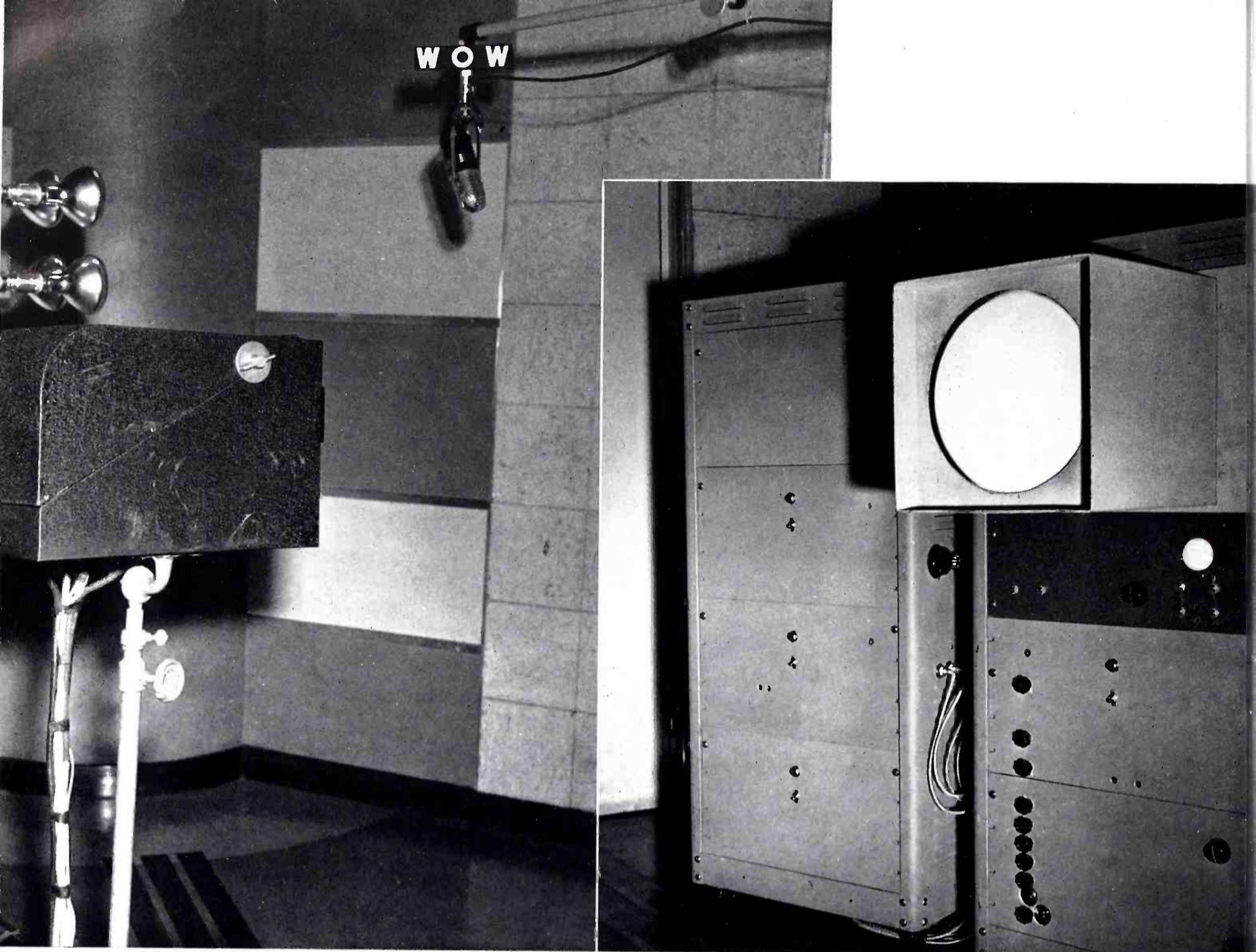
FIG. 1. *WOW* began its television program several years ago with equipment built by the staff. At left above is shown the iconoscope camera and, at right, the camera control and monitor units built by the *WOW* engineering staff.
