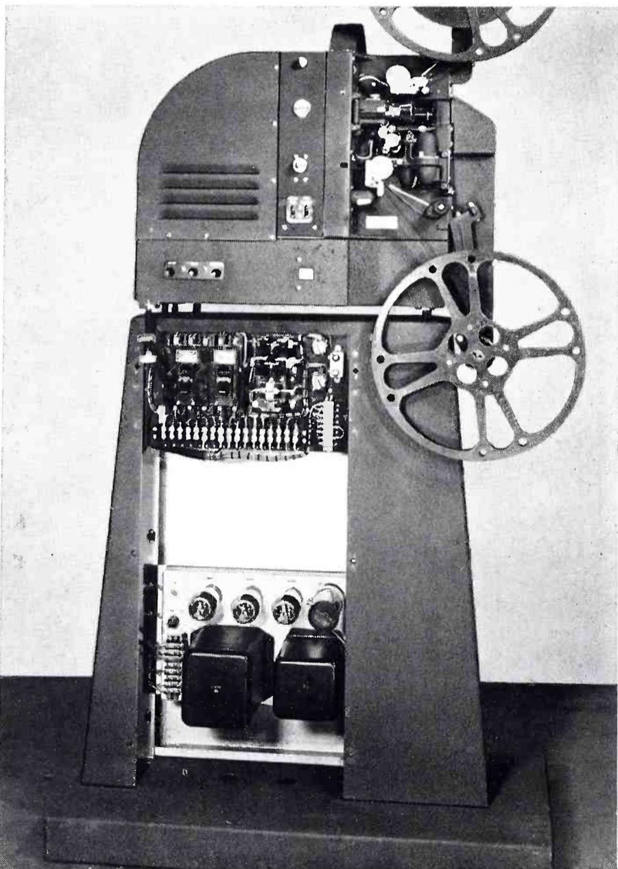
**FIG. 6.** Pedestal covers are easily removed for servicing. Removing the right side cover, as shown here, provides access to the relay panel and field power supply.
