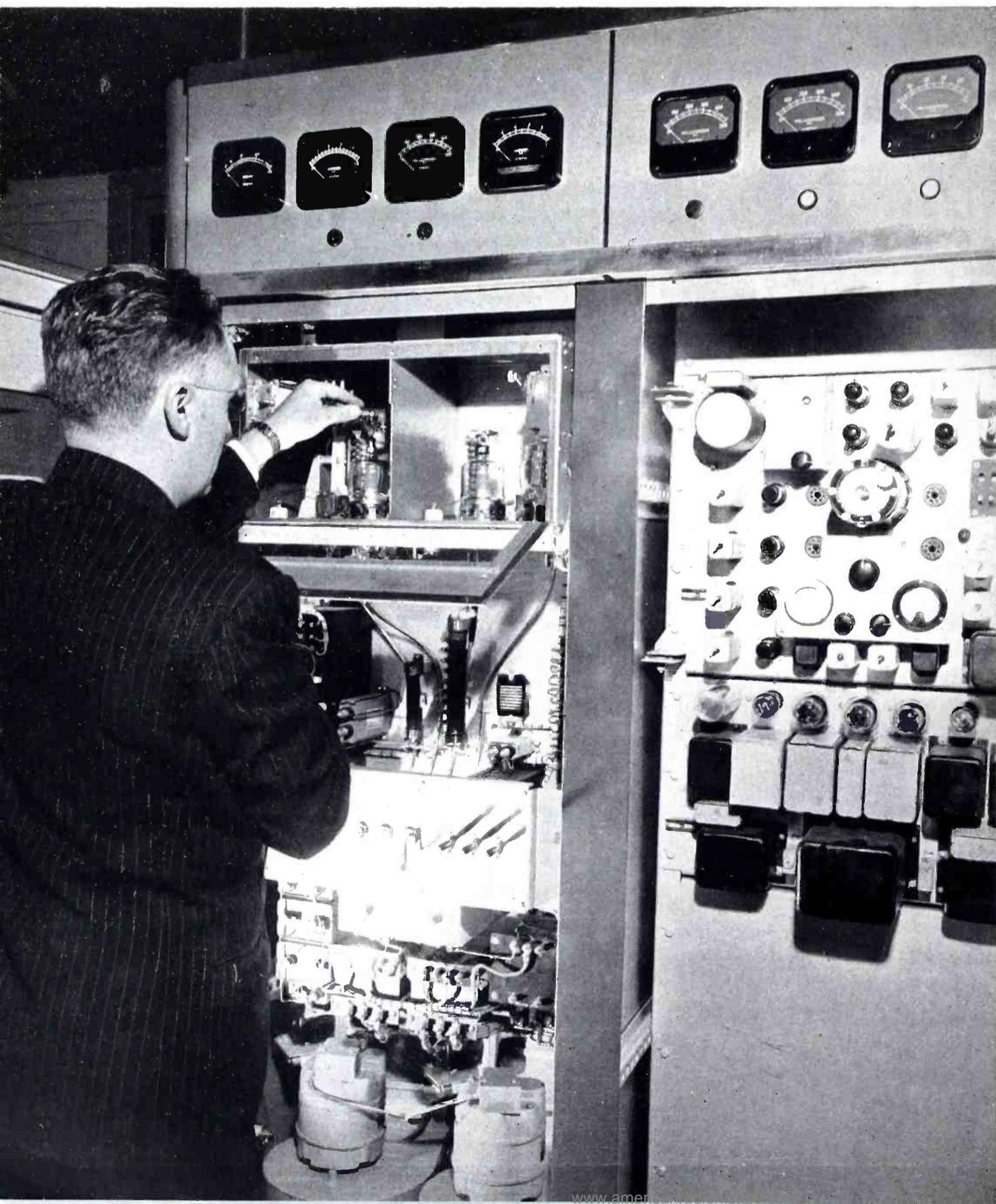
FIG. 10. (Left) A partial view, taken during installation, of the 3 kw RCA FM transmitter. Chief Engineer R. A. Isberg is shown holding an anode connector for one of the 250 watt driver tubes just installed. I.P.A. and Final amplifiers are located in the same left hand cabinet. The cabinet at the right houses the direct FM exciter and its power supply. The high-voltage power supply and control circuits are in the extreme right-hand cabinet (not shown in this view).
