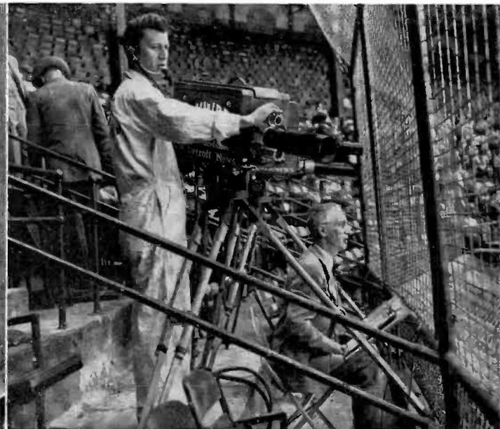
WWDT, Detroit (Tigers) uses two RCA TK-30A Cameras. Both are at the same location, in the lower stands just behind homeplate. Since the pictures above were made, shatter-proof glass has been substituted for the section of the screen which the cameras shoot through. Using two cameras, the 90MM and 135MM lenses are used for general coverage, with the 15" and 17" lens used for closeups.
