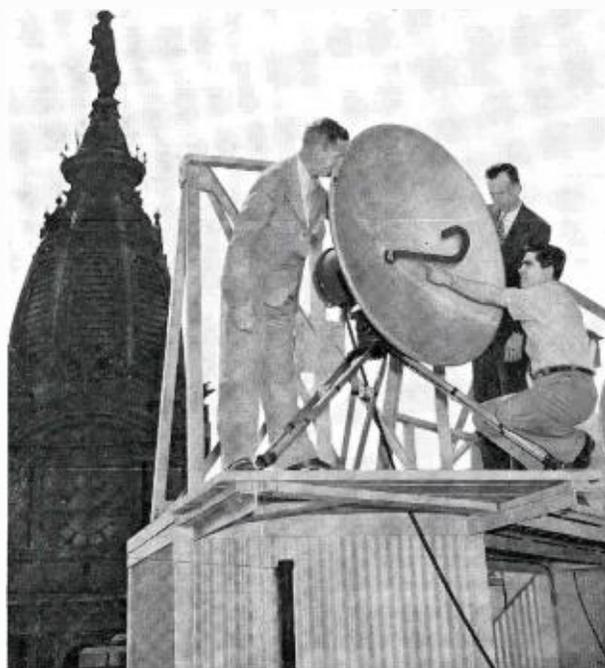
FIG. 1. Receiver antenna mounted on top of 18-story Bank Building in downtown Philadelphia. S. H. Barbour (kneeling) is explaining operation to George E. Hogerty (left), engineering manager of Westinghouse Radio Stations, and W. H. Hauser, Chief Engineer of WBZ.
