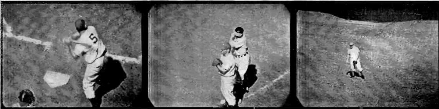
430MM (17") lens was in use on No. 2 camera (behind home-plate, 60 feet high) when the three pictures above were made. This lens, with its narrow (4 degree) angle, is used regularly by some stations to provide a closeup of the batter (left, above) on the "3-and-2" pitch. It is used by most stations to
