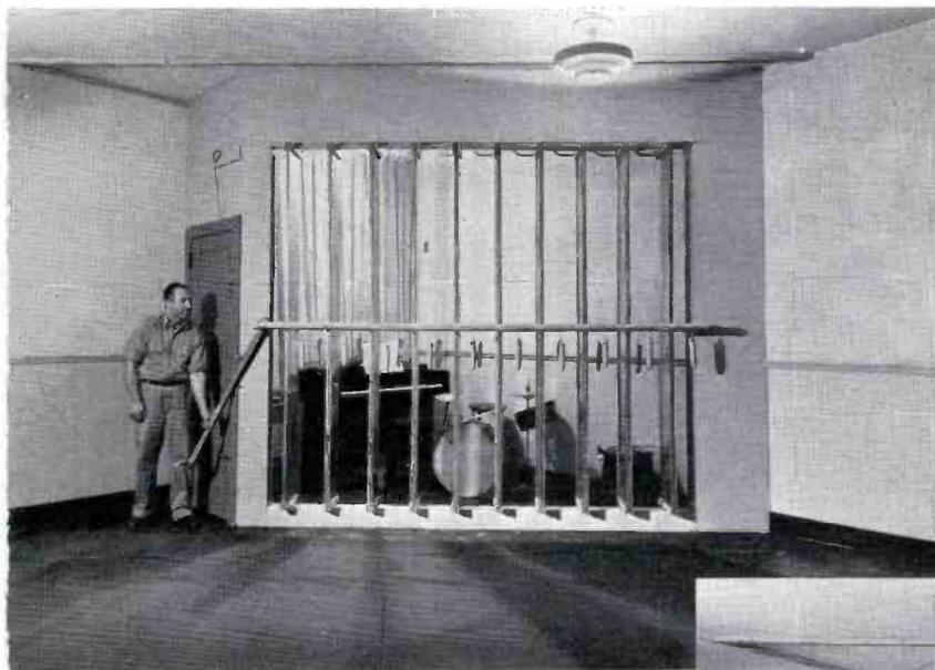
FIG. 4. (left) The acoustical filter consists of eight vanes each 1 foot wide by 8 feet high. These are pivoted at top and bottom so that the whole group can be turned in or out by operation of the lever as shown here.
