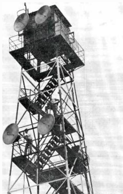
FIG. 2. Transmitter antenna (the parabola at lower left) mounted on Western Union Relay System tower at Bordentown, N. J., about 27 airline miles from the receiving antenna.
