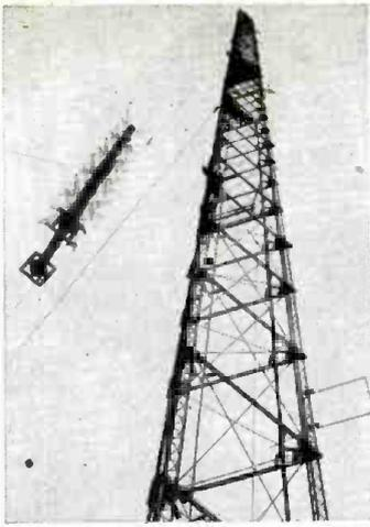
**TWO-AND-A-HALF-TON, 75-foot, five-bay super turnstile television antenna is hoisted to top of WKY-TV Oklahoma City tower. Eight workmen did the hazardous job, WKY-TV reports. Overall tower height is 968 feet.**
