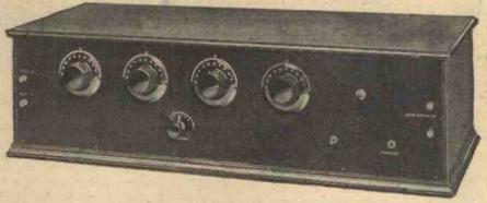
Anode bend rectification is employed in the "Remarkable Five-Valve Receiver," with which loud-speaker results of excellent quality have been obtained from a large number of broadcasting stations.
