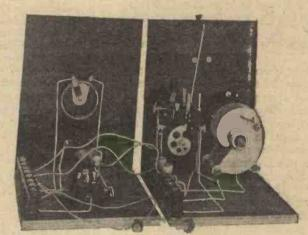
the tuner panel A, the valve detector panel B, and the first-stage L.F. amplifier panel C. arrangement may of course be emploved with or without reaction, and should give full loud-speaker strength on local signals.
