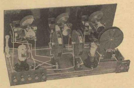
The two coils shown parallel to each other are the ones forming the H.F. transformer. For good selectivity they will usually require to be placed almost at right angles.
